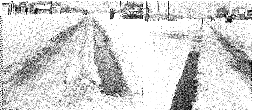
FIGURE 4. BITUMINOUS PAVEMENT 12-18-51 LOOKING EAST. INSIDE TRACK CLEAR, OUTSIDE TRACK COVERED WITH SLUSH.
