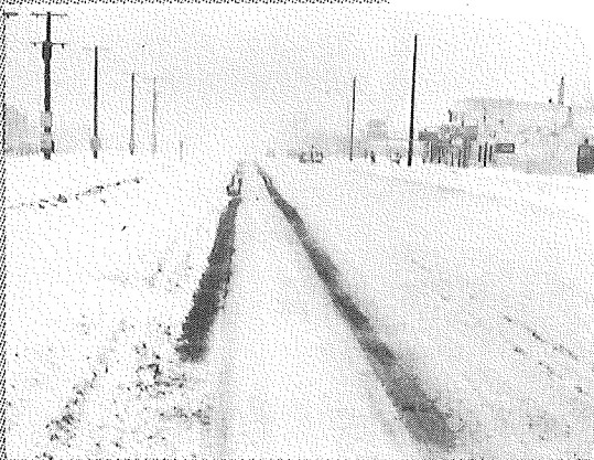
FIGURE 5. CONCRETE PAVEMENT 12-20-51 SHOWING CONDITION OF HEATED SECTIONS.
