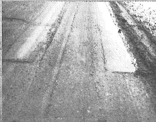
FIGURE 7. CONCRETE PAVEMENT 2-20-52 SHOWING CONDITION OF HEATED SURFACE.
