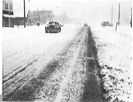
FIGURE 6. BITUMINOUS PAVEMENT 12-20-51 SHOWING CONDITION OF HEATED SECTIONS.
