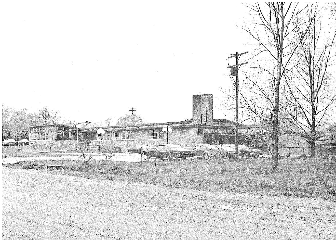
Figure 22. Microphone located 10 ft from E side of Kurtz Elementary School. Observer looking NW. Sta. 654.
