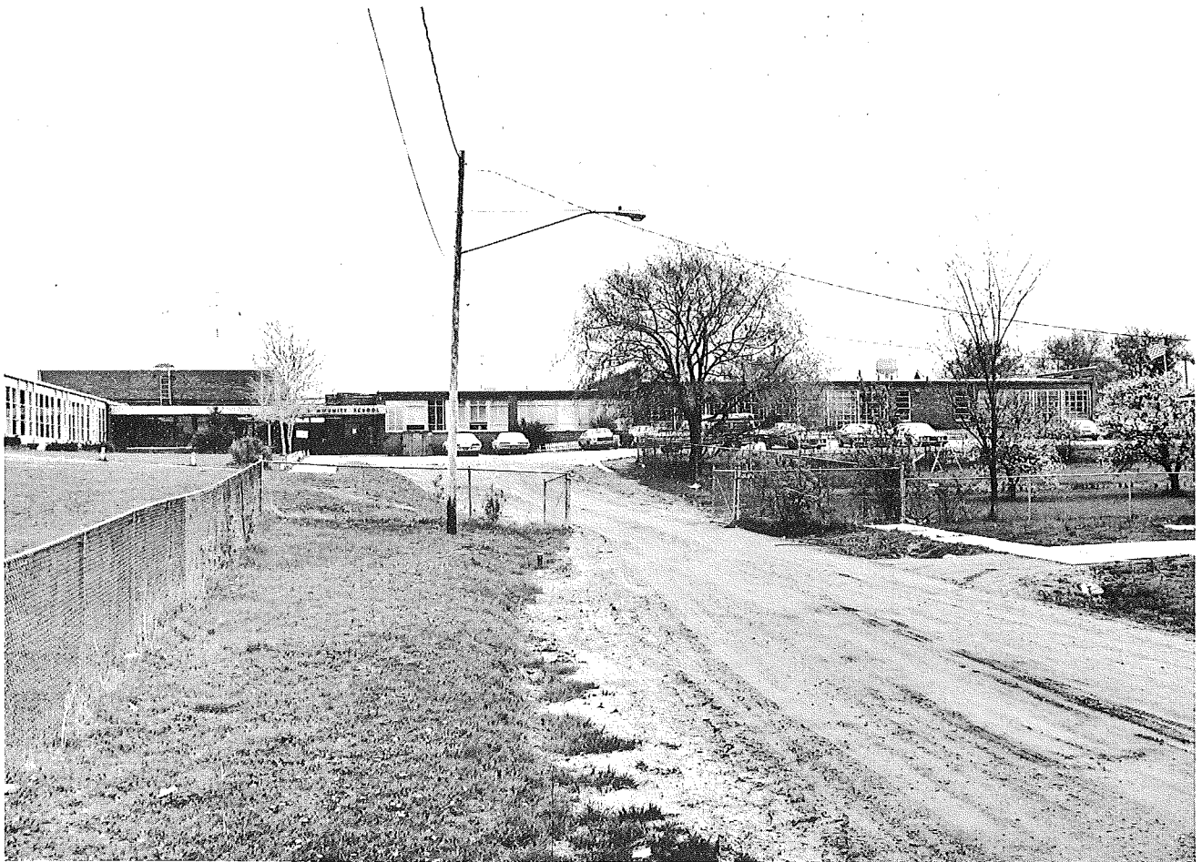
Figure 23. Microphone located 15 ft from W part of Buick Community School. Observer looking E. Sta. 688.
