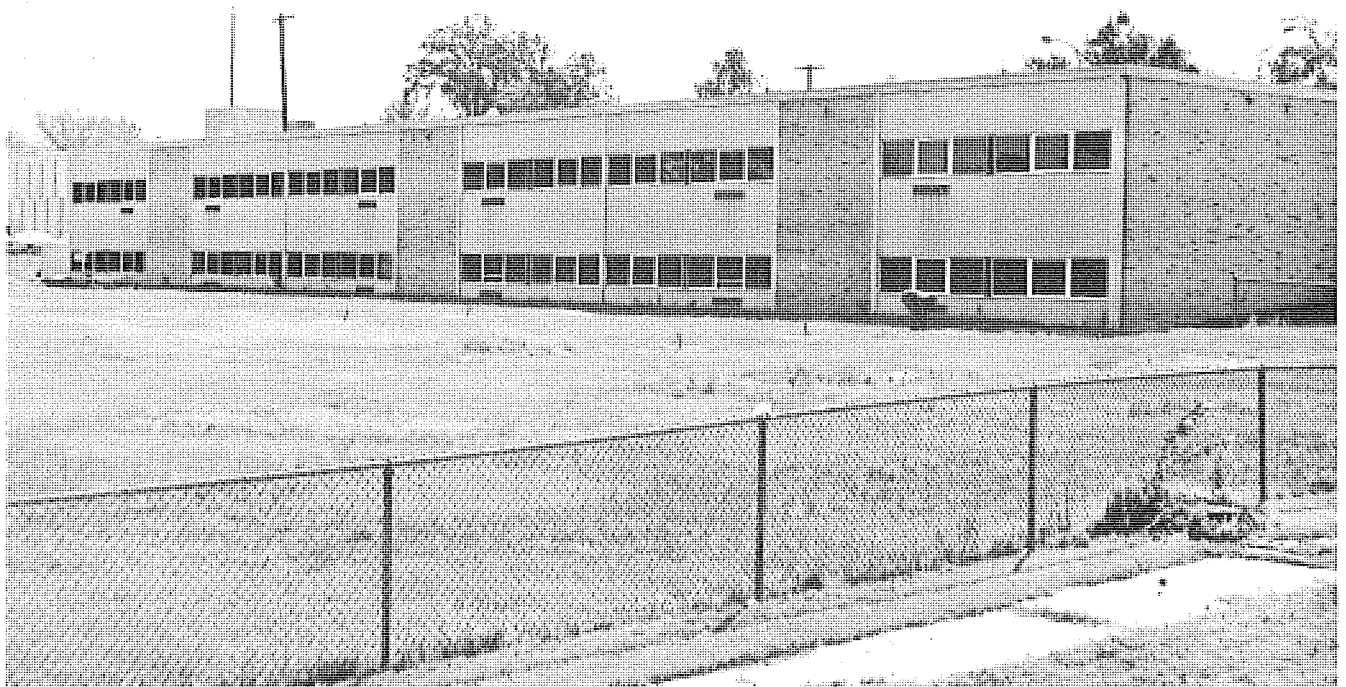
Figure 5. Microphone located on N side of Walker School at the right-of-way. Observer looking SE. Sta. 398.
