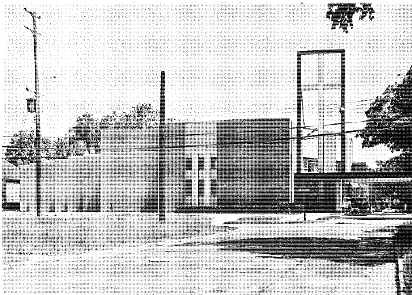
Figure 4. Microphone located on W side of Riverside Assembly of God Church at proposed right-of-way. Observer looking E. Sta. 386+50.
