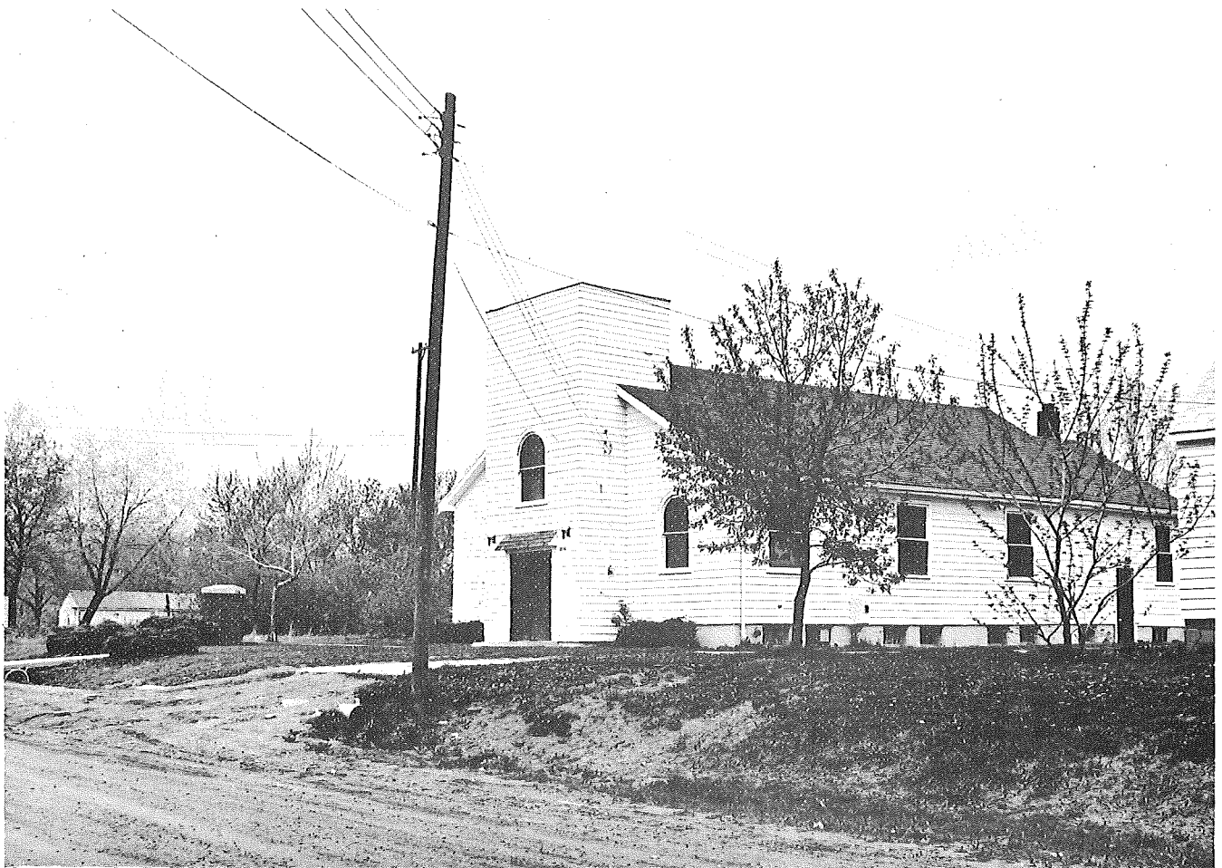
Figure 20. Microphone located 20 ft N of SE corner 6 ft from E wall of Emmanuel Temple Apostolic Church. Observer looking NW. Sta. 632.
