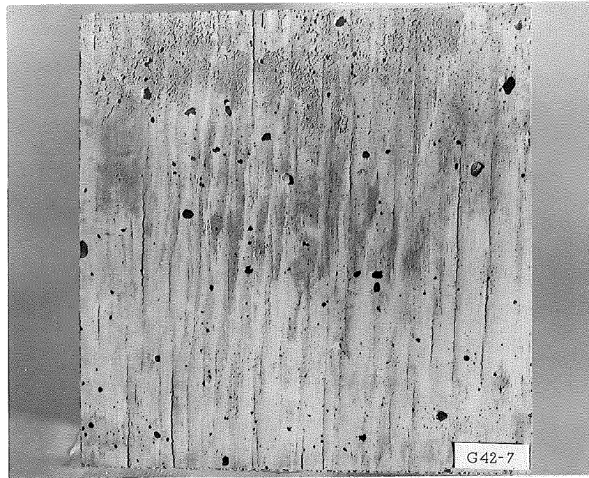
Figure 4. Surface showing effect of warping and cracking of plywood after being used six times.
