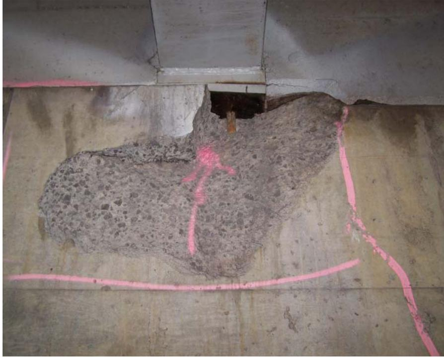
**Figure 1-2 Pull-out of concrete block in the abutment wall of Bridge A 1.7**
