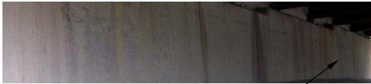
Vertical crack in abutment wall (between girders, amplified in the right figure)
