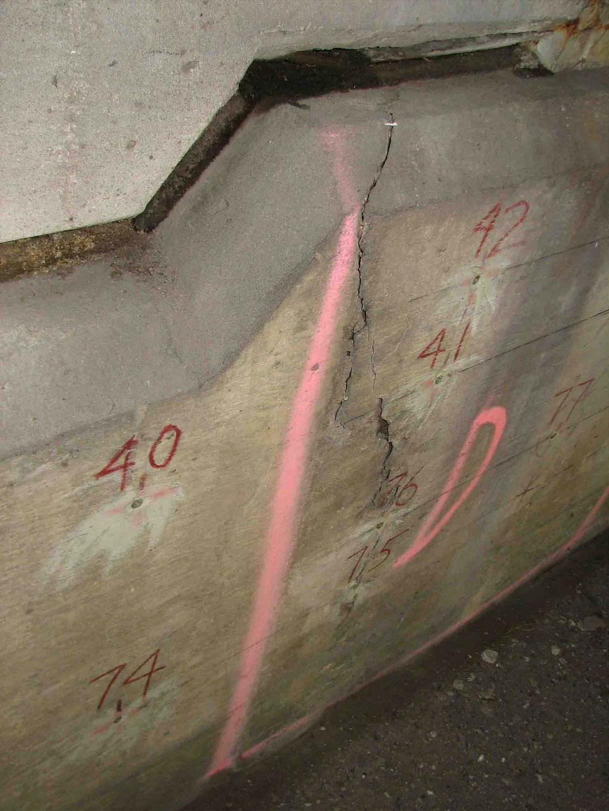
Figure 7-6 Abutment distress in bridge A 1.7
