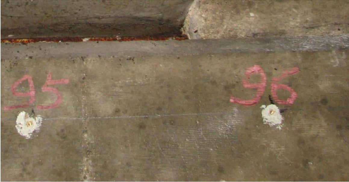
**Figure 4-2 Brass cylinders installed on the abutment wall**
