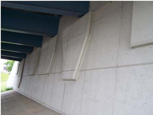
(a) Repaired abutment wall with U – shape patch
