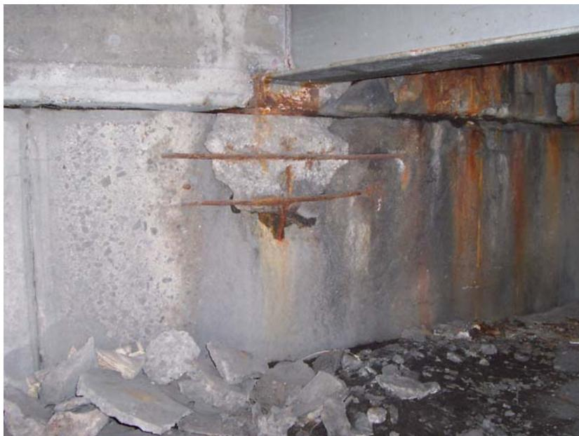
**Figure 1-1 Concrete spalling in the abutment wall of bridge B 2.1**
