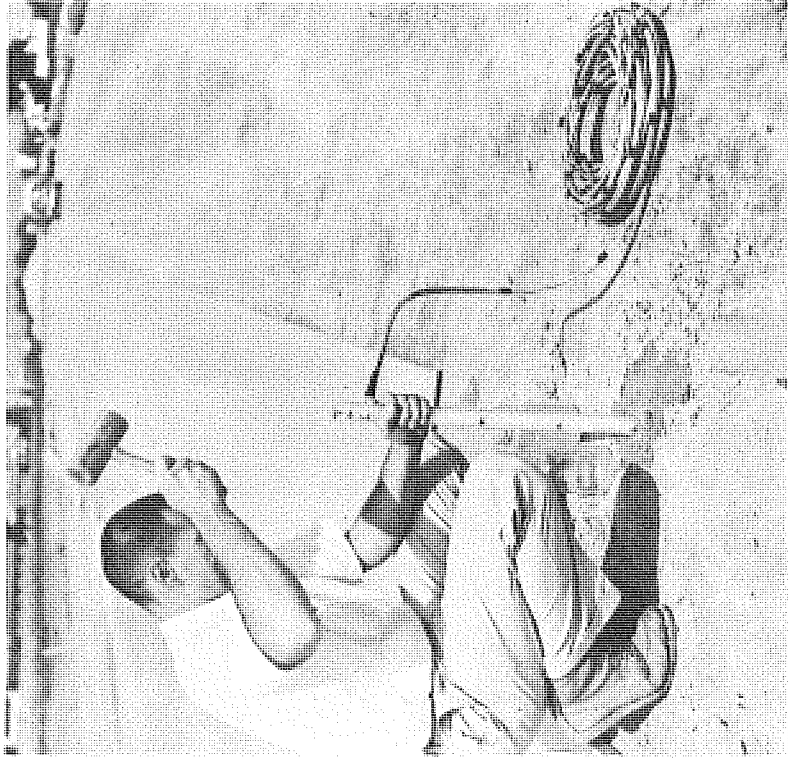
Figure 6. Equipment used in placing thermocouples (upper left), insertion of rod in subgrade (upper right), appearance of installation before covering (lower left), and placement of cables directly on subgrade using U-clips (lower right).
