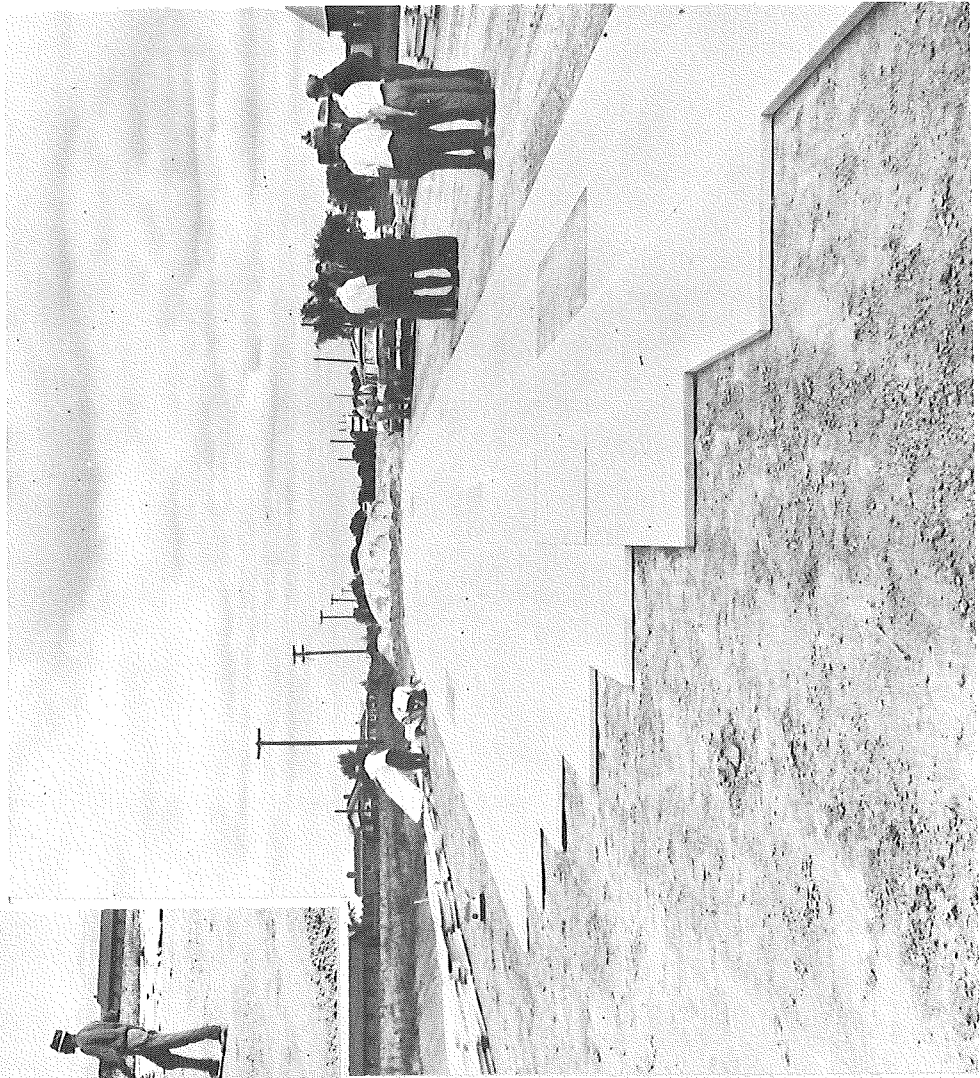
Figure 3. Delivery and placement of Styrofoam.
