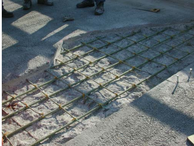
Figure 9.6: Completed patch repair preparation
