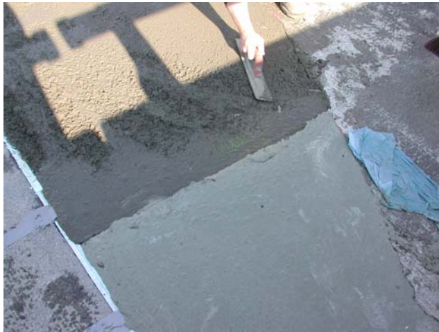
Figure 9.13: Comparison of HES-ECC patch repair and Thoroc 10-60 patch repair
