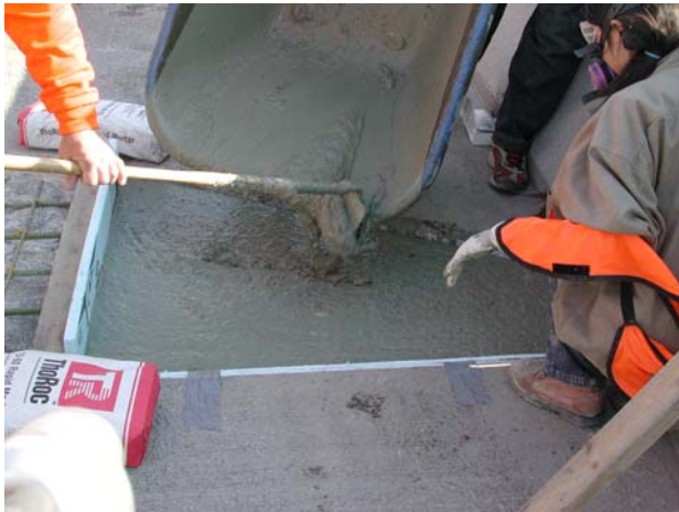
Figure 9.10: HES-ECC was poured into patch
