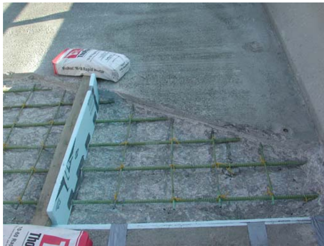
Figure 9.7: Separated patch areas for HES-ECC repair and Thoroc 10-60 repair
