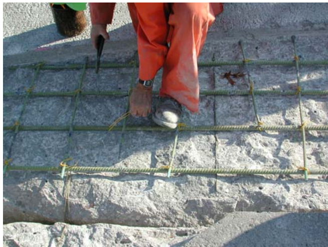
Figure 9.5: Replacement of damaged reinforcement
