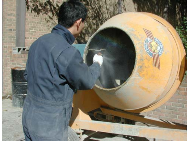
a) Pre-wetting the mixer
