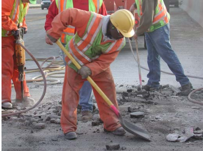
Figure 9.3: Partial depth removal
