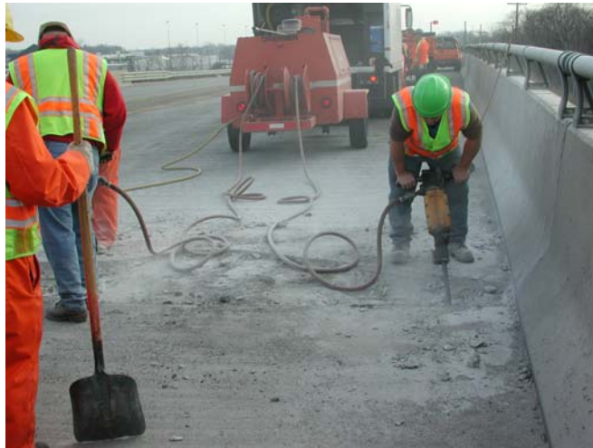
Figure 9.4: Sandblasting of patch area
