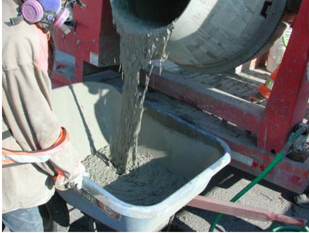
Figure 9.9: Pouring HES-ECC into wheelbarrow for transportation
