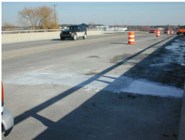
Figure 9.14: Completed patch repair work
