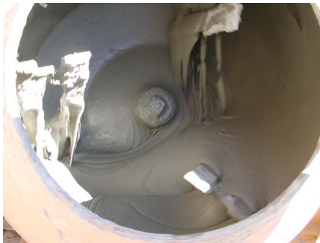
c) After adding cement (homogenous and creamy HES-ECC mortar matrix)
