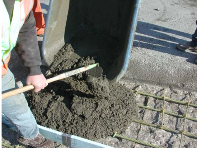
Figure 9.12: Placement of Thoroc 10-60
