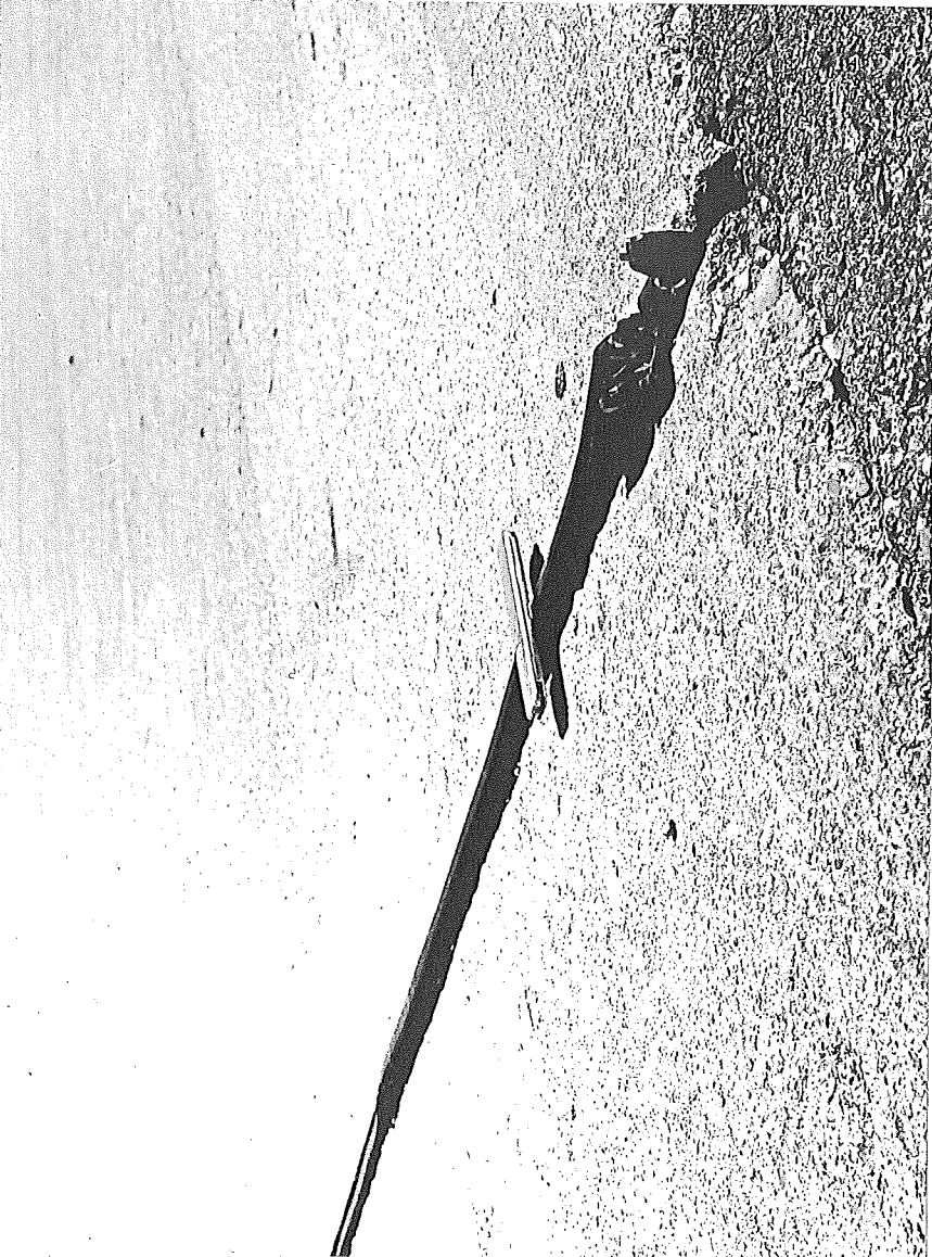
Figure 1. Expansion seal with end partially expelled from joint, which is closed to 1/2 in. at this point.
