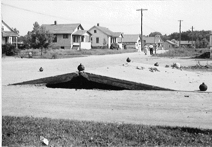
B. Compressive Failure manifested by sudden eruption of a large section of pavement. 5-39F-7 (6B)
