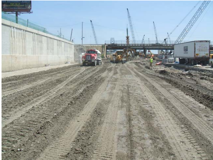
Figure 7: Grading
