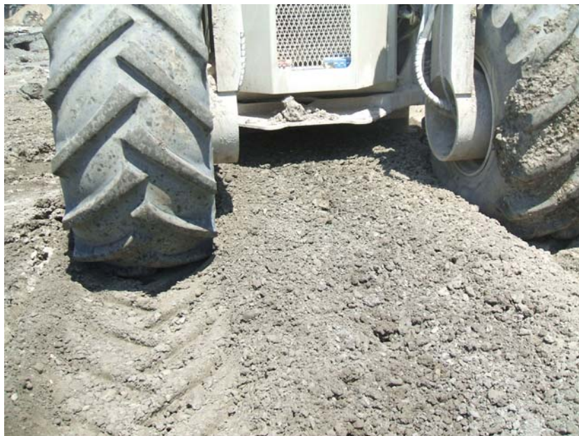
Figure 4: Mixing with Rotary Pulverizer
