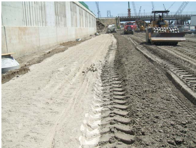
Figure 8: Finishing Different Areas of Test Area 1
