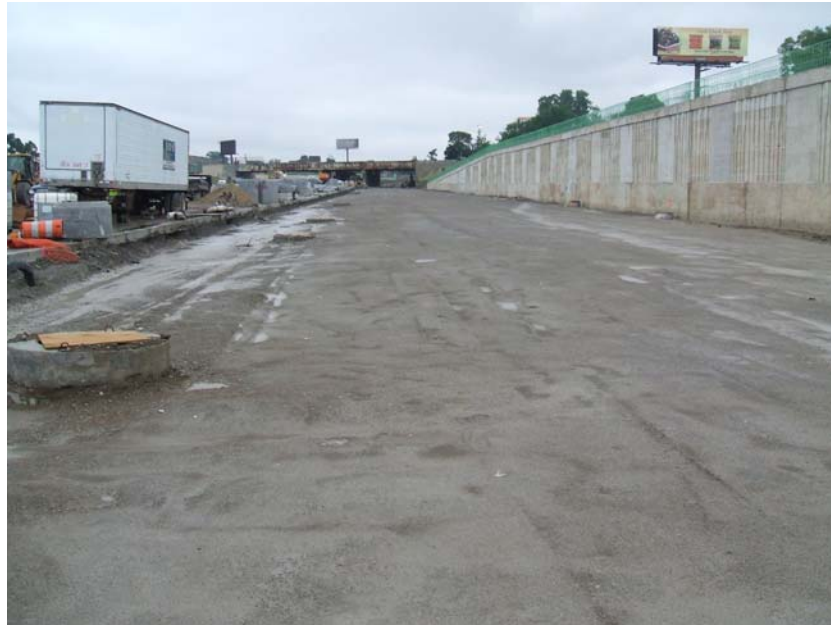
Figure 9: Finished Grade of Test Area 1
