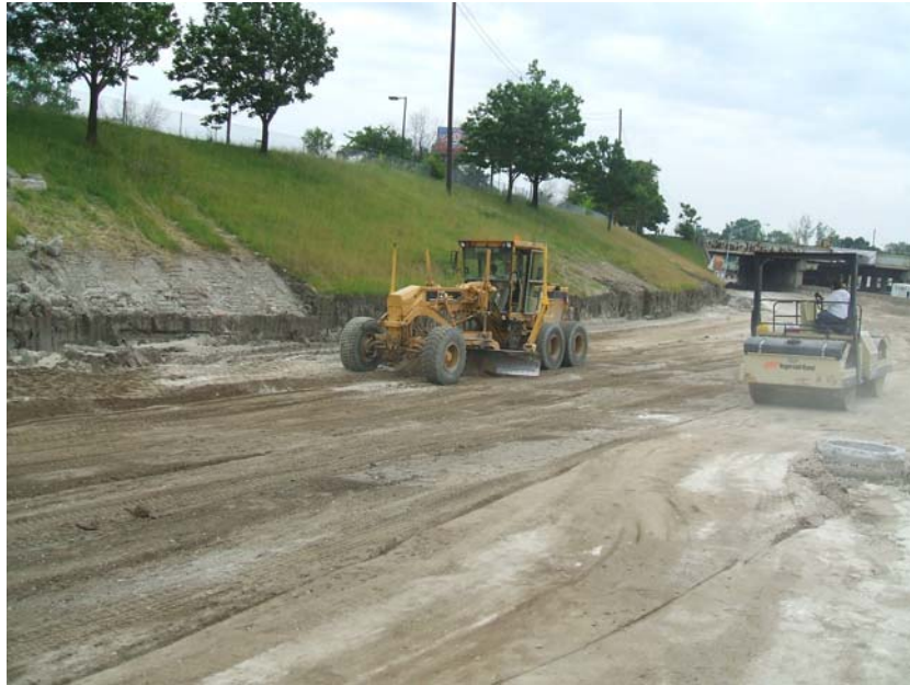
Figure 14: Final Rolling with Smooth Roller and Final Grading
