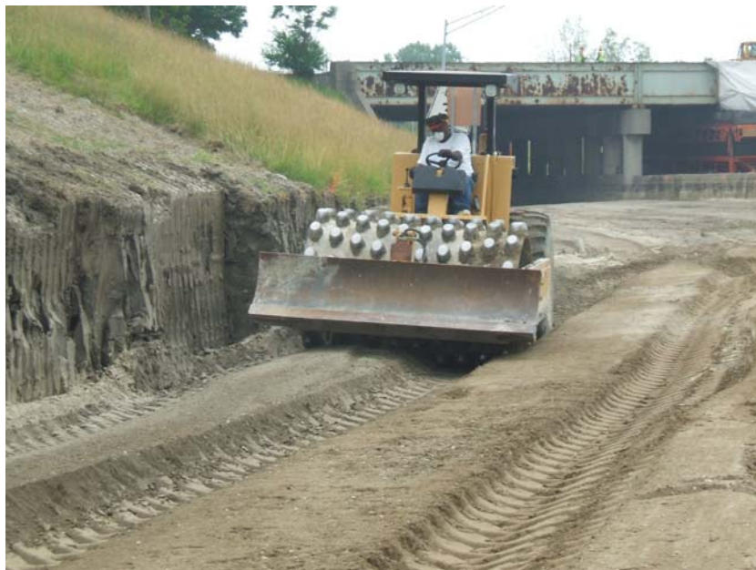
Figure 13: Rolling with Sheep Foot Roller
