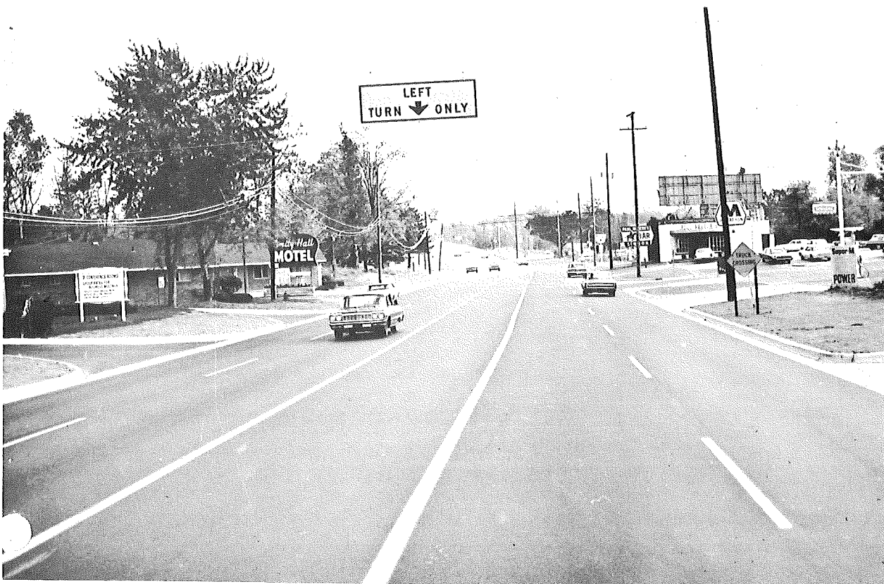
Typical 5-Lane Roadway in the After Period
