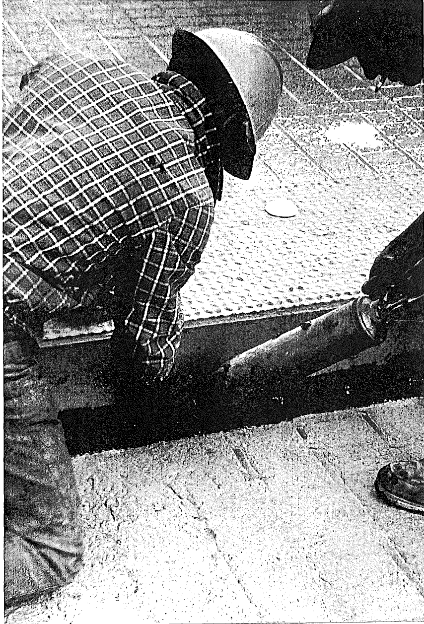
Figure 3. Sealing median curb joint with 2.5-quart caulking gun.
