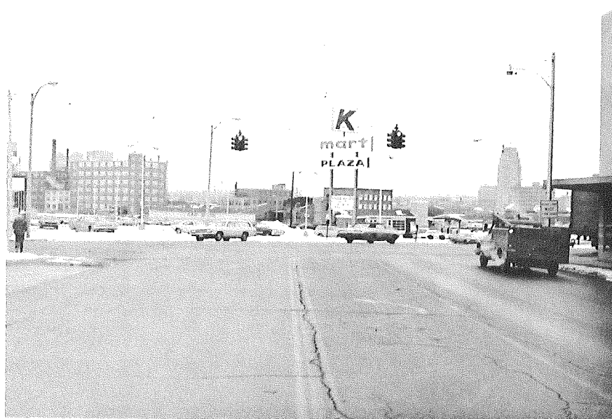
NORTHEASTBOUND CAPITAL AVENUE
