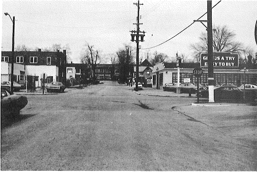
NORTHBOUND CASS STREET
