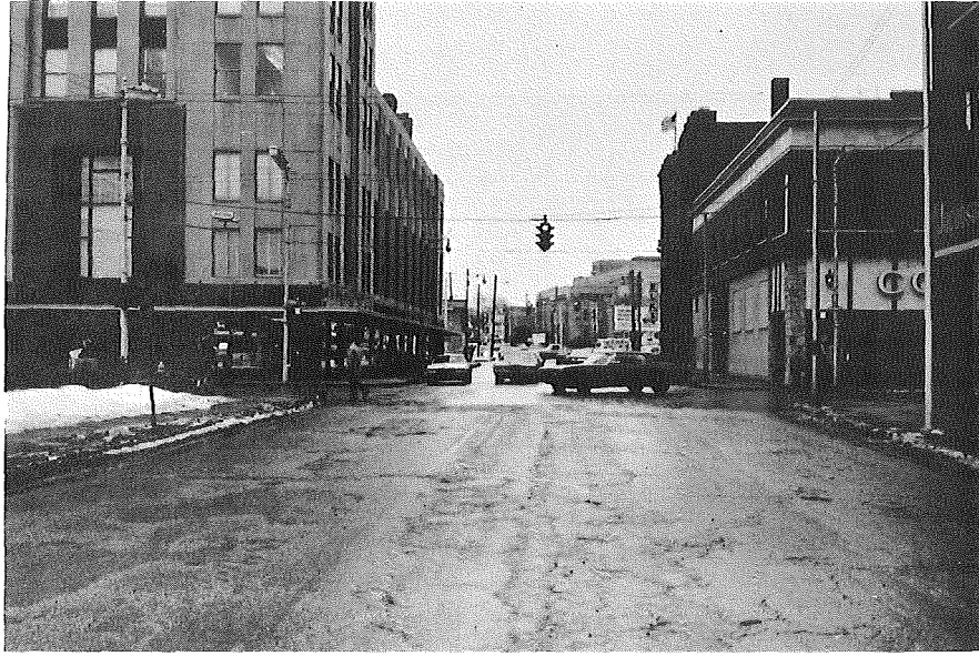
NORTHBOUND McCAMLY STREET
