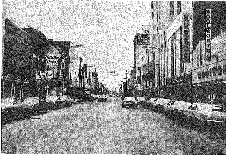
EASTBOUND MICHIGAN AVENUE AT CROSSWALK
