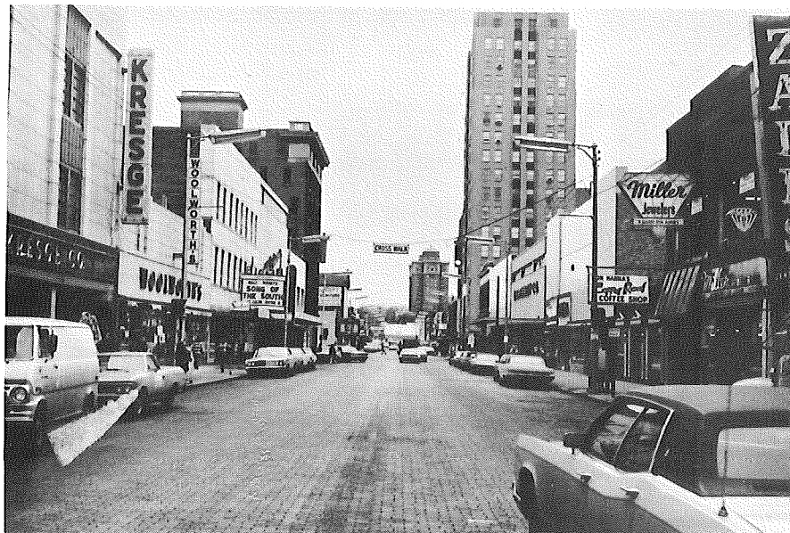
WESTBOUND MICHIGAN AVENUE AT CROSSWALK
