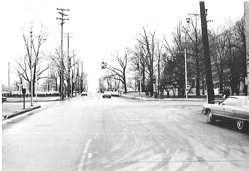
NORTHBOUND WASHINGTON AVENUE
