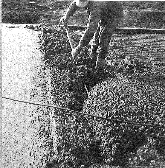
▲ FIGURE 5. PLACING CONCRETE AROUND JOINT SEAL.
