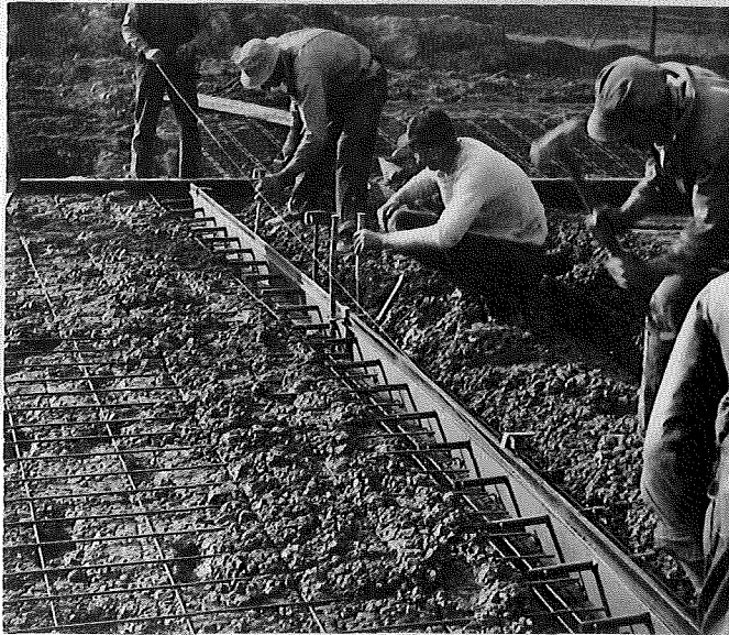
▲ FIGURE 3. STAKING ASSEMBLED JOINT IN PLACE.
