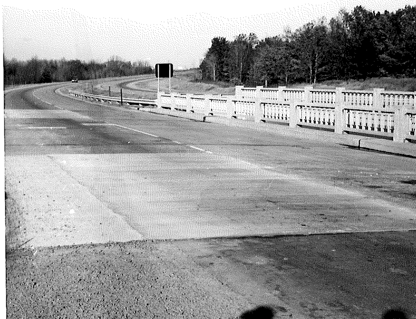
Figure 7. Latex concrete patches placed 8-23-68 in southbound US 127 over the Grand River (11-13-68).
