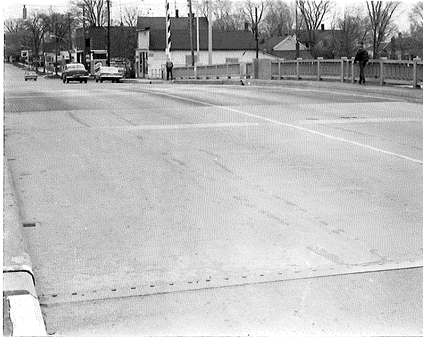
Figure 1. Latex mortar surfacing on west end span, looking east on US 23.
