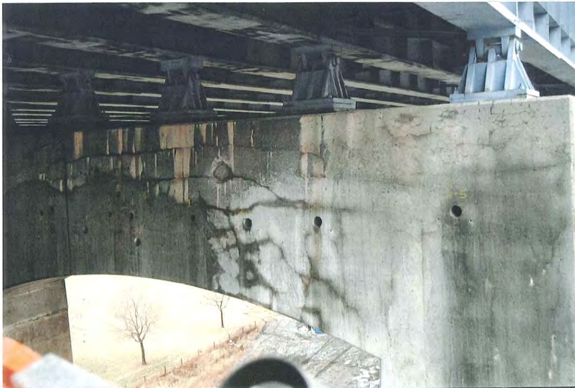
Figure 11. South face of Pier 39 north-bound showing locations of cores. One additional core was taken in the column at the right side of the photo.
