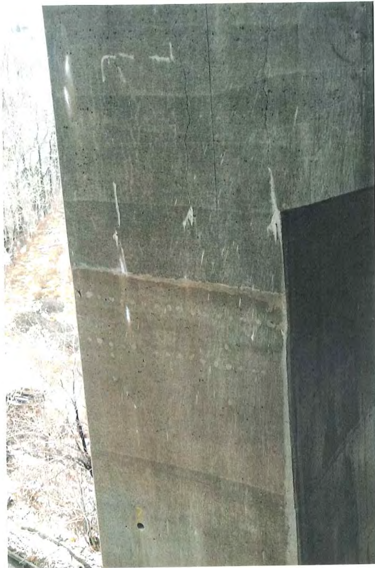
Figure 4. North face of Pier 38 north-bound and outer column. Note the difference in color between the pier cap and column.
