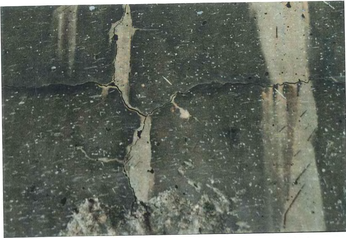
Figure 6. Close-up of south face of Pier 39 north-bound showing the typical pattern cracking seen on the pier caps.
