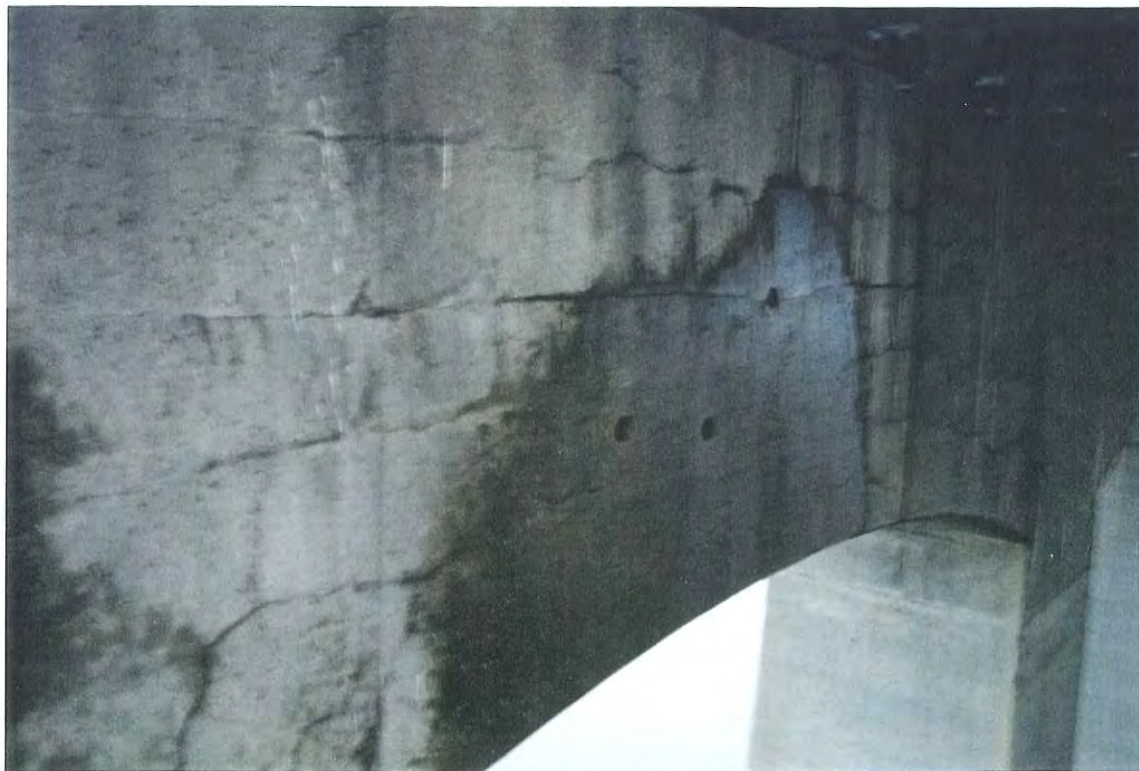
Figure 13. South Face of Pier 38 south-bound, showing all three cores.
