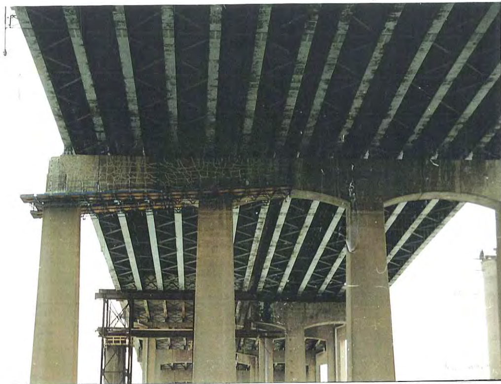
Figure 8. South face of Pier 39 south-bound. The cracks have been injected with epoxy as part of the repair procedure. The left end of the pier cap has been prepared for post-tensioning.
