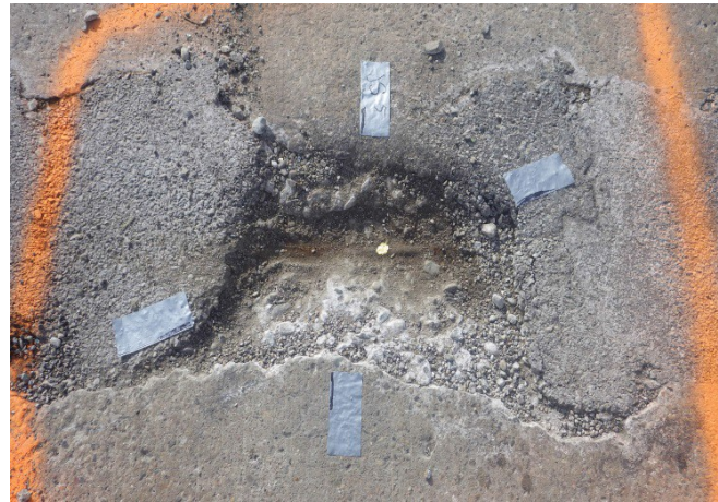
Figure 12: Manual measurements the length, width, and depth of spall and patch features on the bridge deck.
