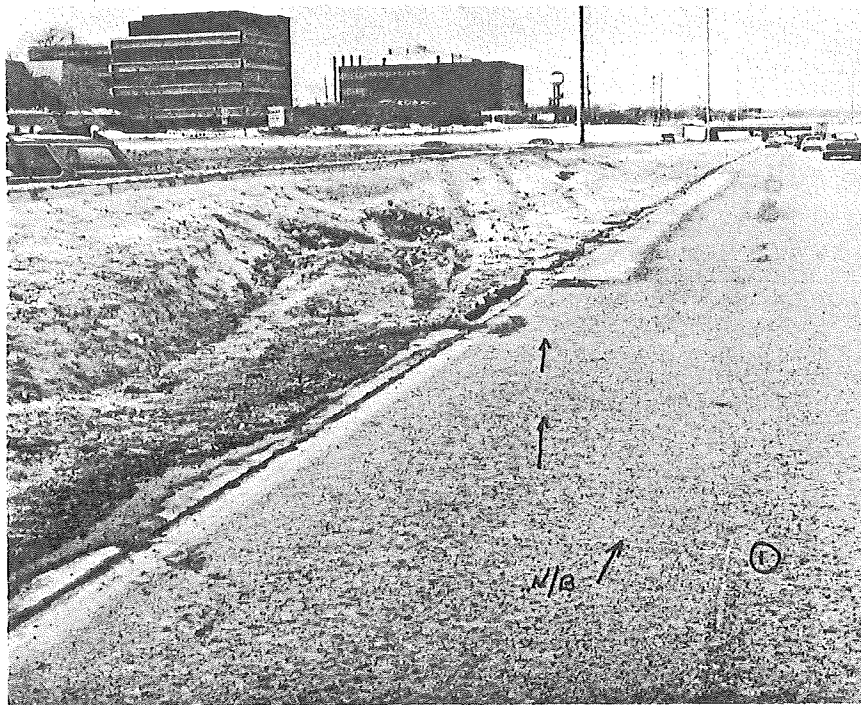
Figure 3. Photo shows where vehicle mounted snow wedged ramp.
