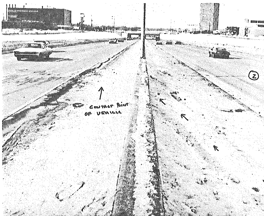
Figure 4. Photo shows contact point after vehicle hurdled barrier.
