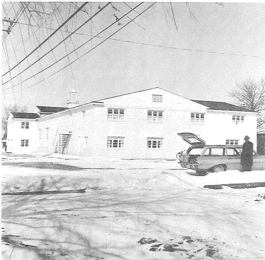
Figure 12. First Baptist Church at 9-1/2 Mile Rd and Coolidge Rd, Oak Park, a cement block structure brush-coated with Gun-Tex 000-SMOOTH in a single coat by members of the congregation in September 1960 at the rate of 50 sq ft per gal. Applicators were unskilled and some were 14-year-old children. General appearance good after two winters. Brown spot bleeding through coating on rear wall was explained by manufacturer's representative as due to insufficient coverage by amateur painters (photos: 3-1-62).
