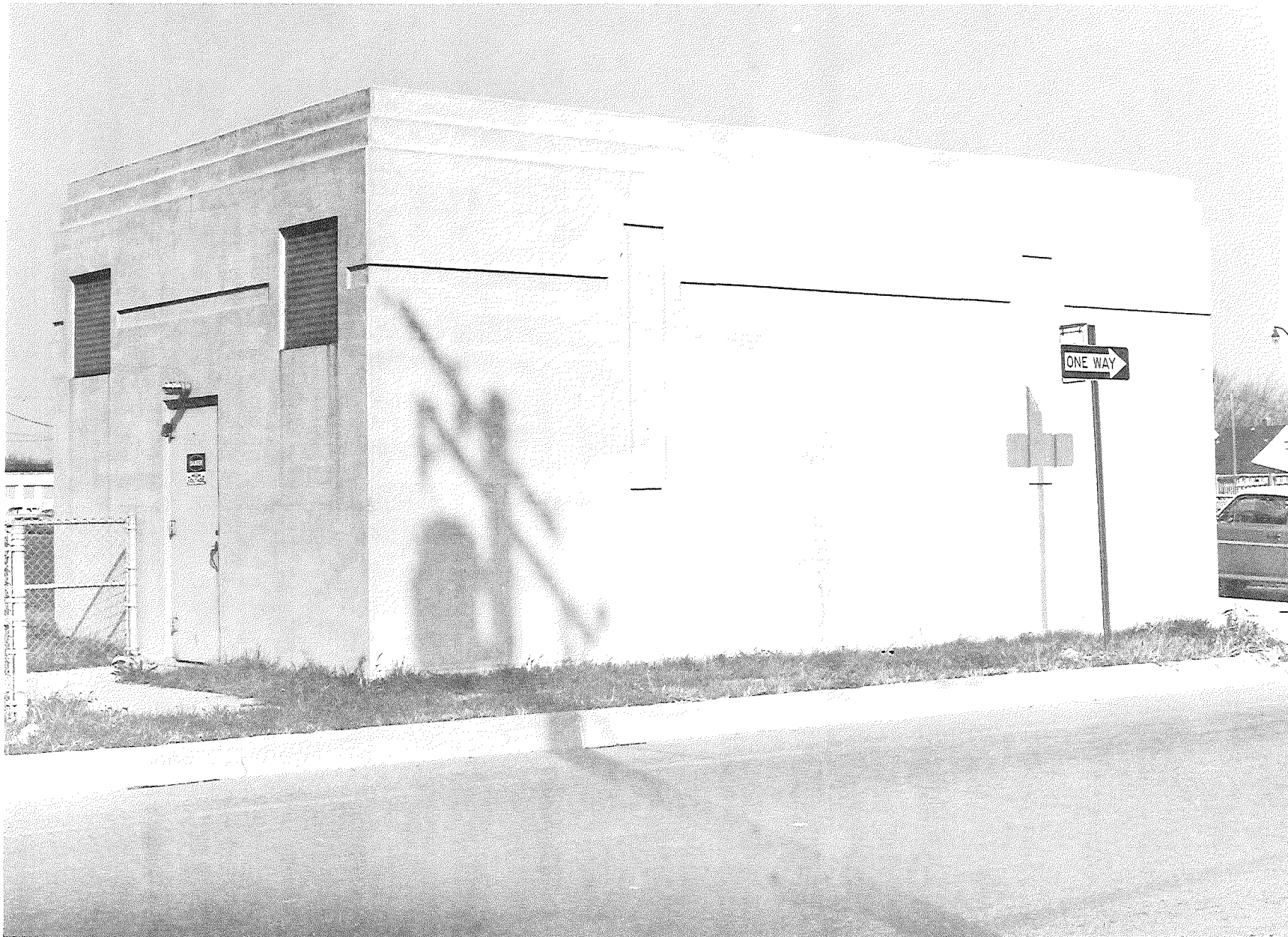
Figure 1. Regulator house with surface finished by hand rubbing, at the Edsel Ford Expressway and Cadieux Ave., Detroit (photo: 11-6-62).
