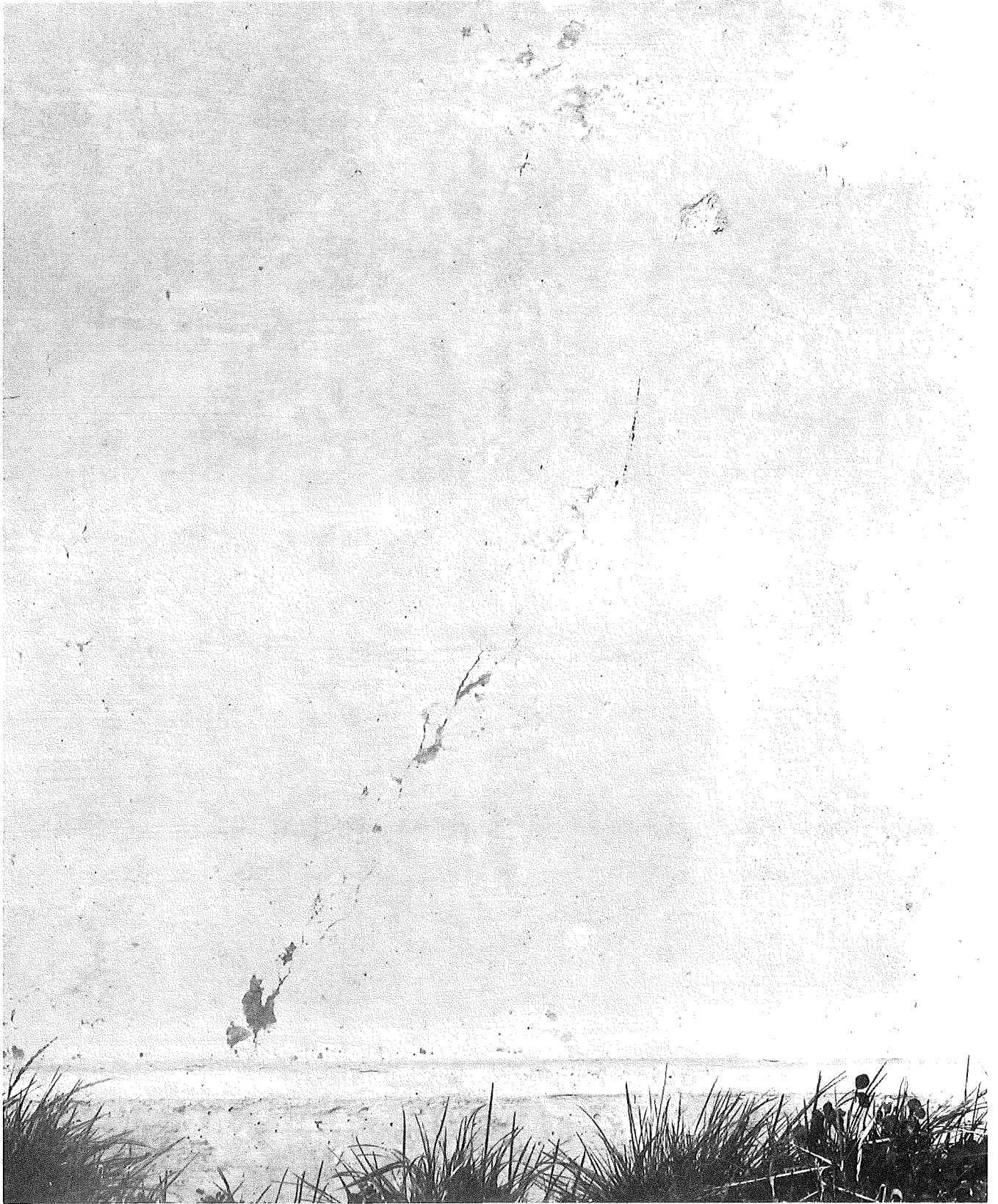
Figure 5. Hand-rubbed finish with typical crack on Cadieux Ave. regulator house (photo: 11-6-62).
