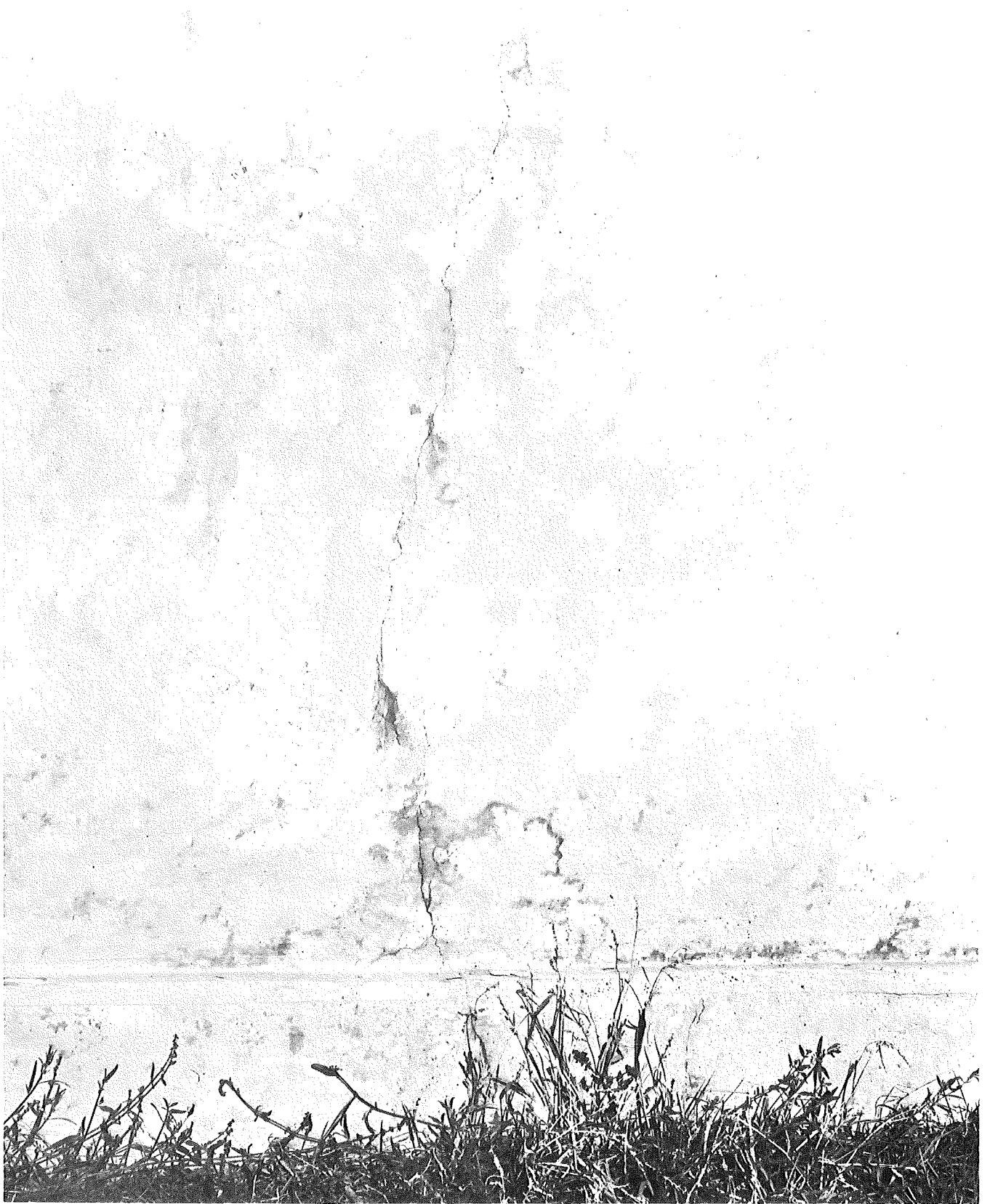
Figure 6. Armor Speed Finish with typical crack on Outer Drive regulator house (photo: 11-6-62).
