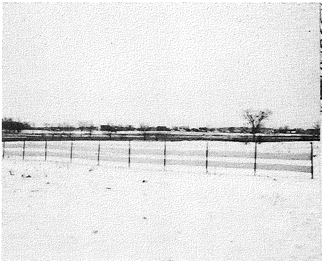
▲ Figure 43. Ten-foot spacing of posts. 1-12-53.
