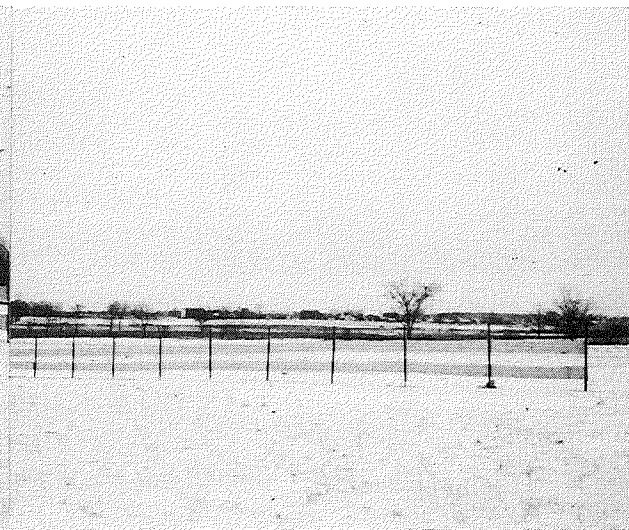
▲ Figure 42. Nine-foot spacing of posts. 1-12-53.
