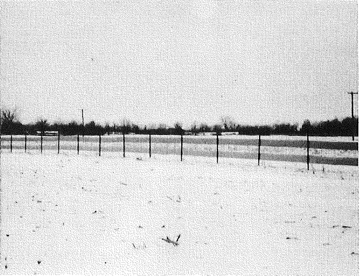
▲ Figure 36. Fence posts spaced 9 feet apart. 1-12-53.
