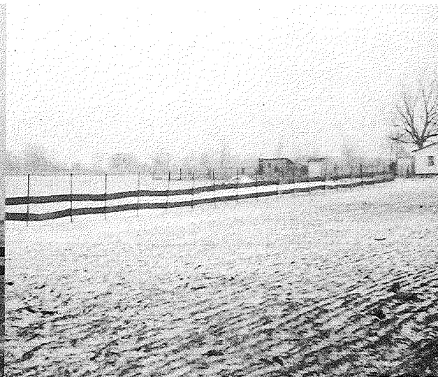
▲ Figure 10. Hillsdale Co. on M-99 detour south of Homer. Note general slackness of paper. 2-11-53.
