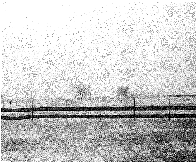
▲ Figure 9. Macomb Co., M-53 south of Romeo. Note slackness in end panel. 1-9-53.
