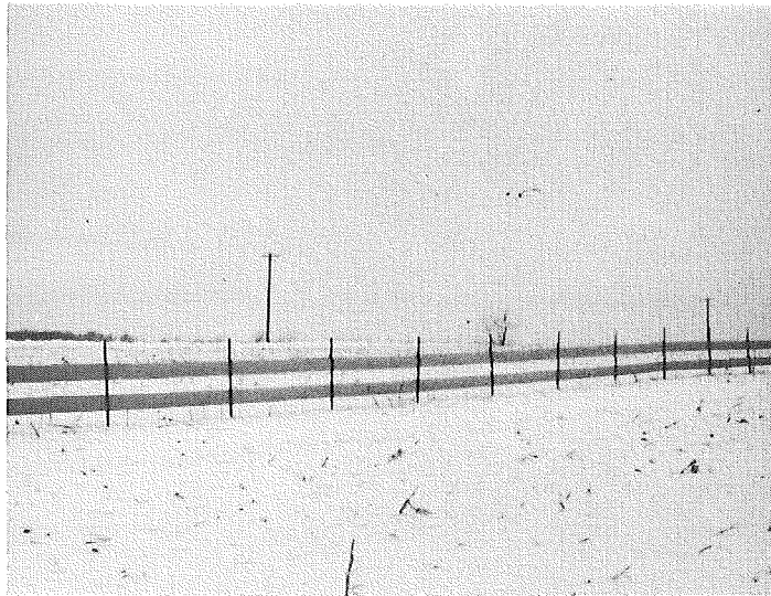
▲ Figure 37. Fence posts spaced 10 feet apart 1-12-53.
