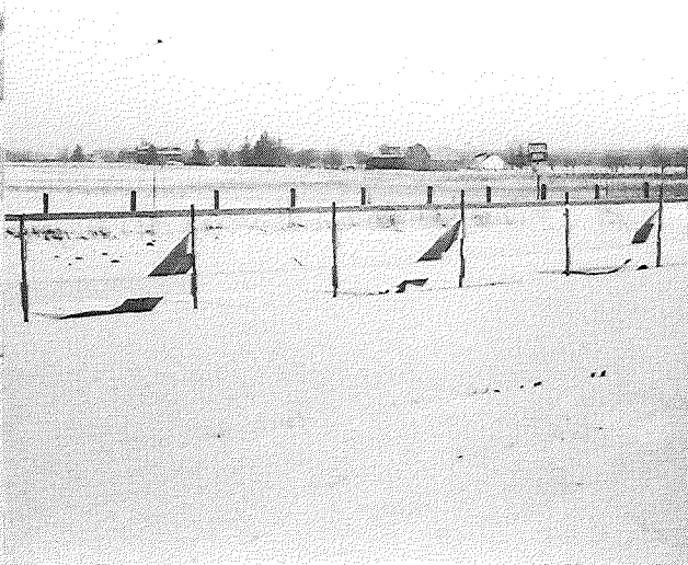
▲ Figure 16. US-131 in Oceana County. Breaks caused by children playing, as evidenced by footprints. 2-18-53.
