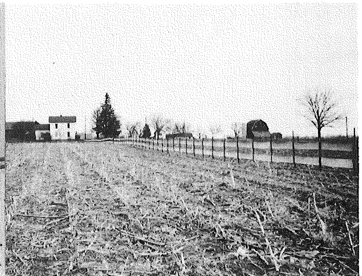
▲ Figure 38. Special installation M-100. General view of snow fence installation. 1-16-53.
