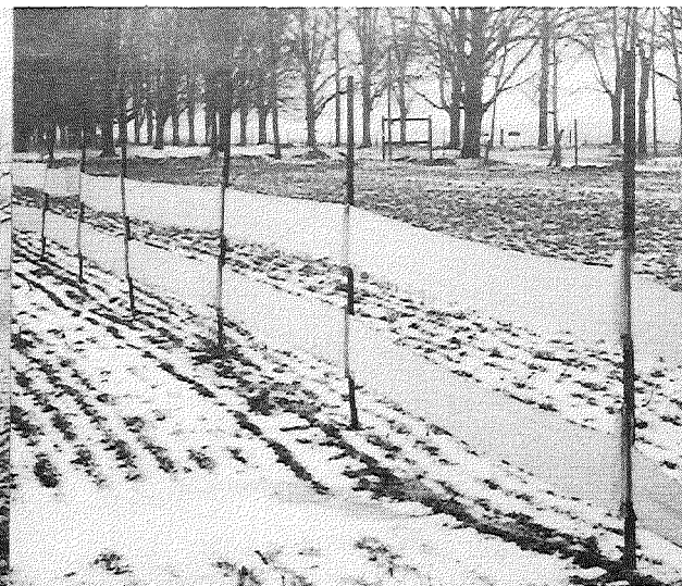
▲ Figure 11. Hillsdale Co., M-99 north of Litchfield. Use of wire bracing. 2-11-53
