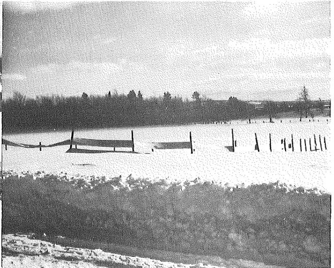
▲ FIGURE 10. CONDITION OF FENCE WHEN IMPROPERLY INSTALLED. IN THIS CASE FENCE POSTS WERE SET TOO FAR APART - 8 FEET WOULD BE THE MAXIMUM SPACING
