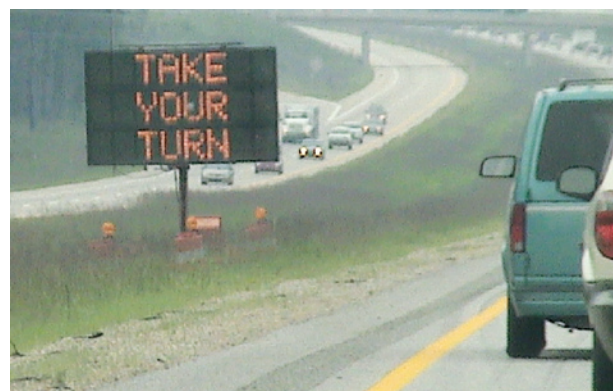
The DLLMS improves traffic flow and safety for vehicles merging in high-congestion work zones.
