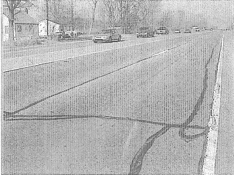
Stations 38+00 - 51+00, NB Lanes Looking North (Polyguard NW-75)
