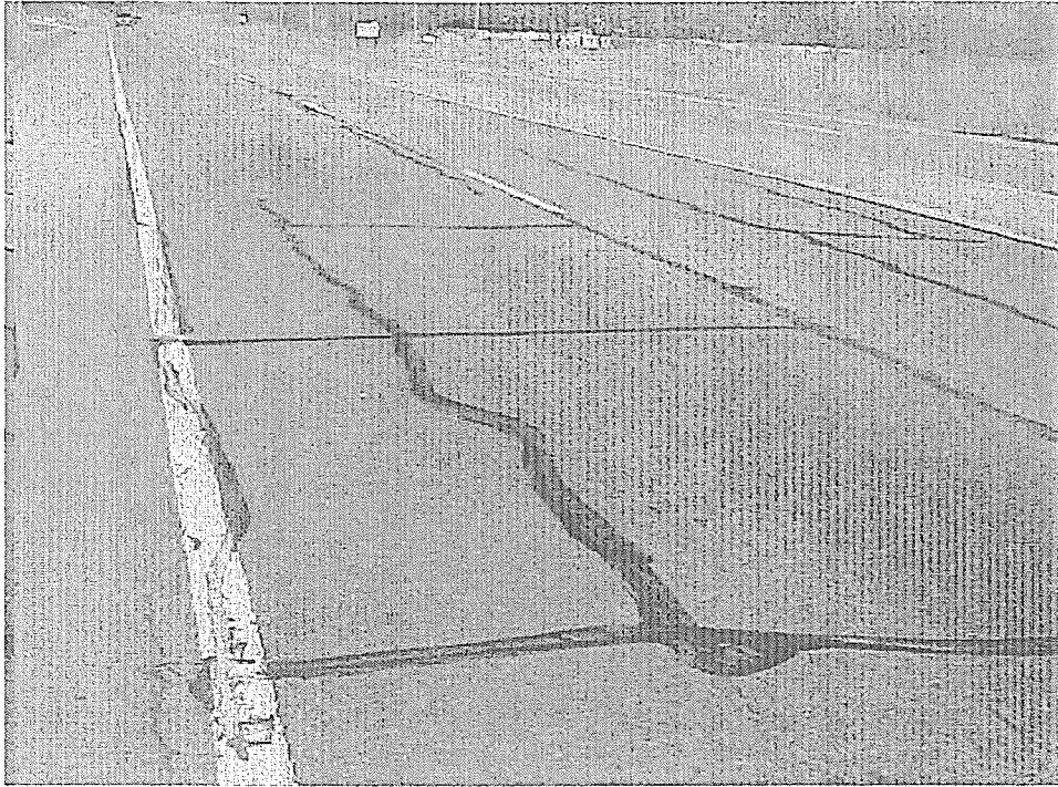
Station 87+25, SB Lanes Looking North (24" Pro-Guard)
