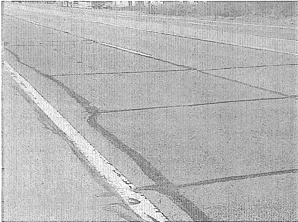
Station 56+00, SB Lanes Looking North (Petrotac)
