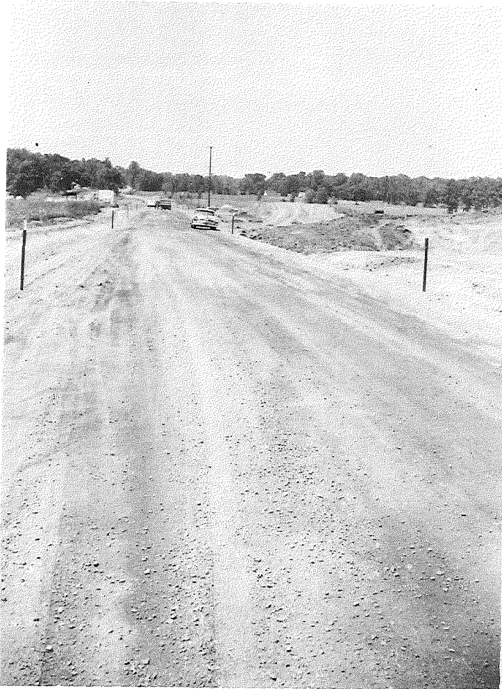
Figure 17. Appearance of liquid chloride treated base course (above).
