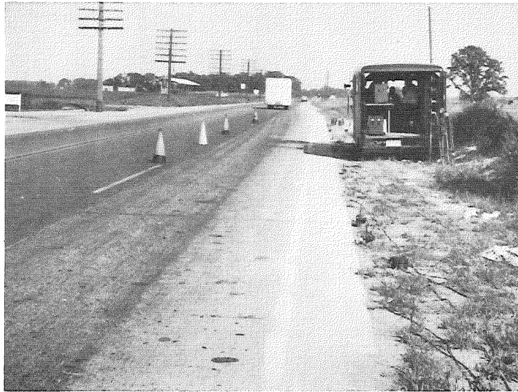
▲ FIGURE 2. SITE FOR PAVEMENT DEFLECTION STUDY.
