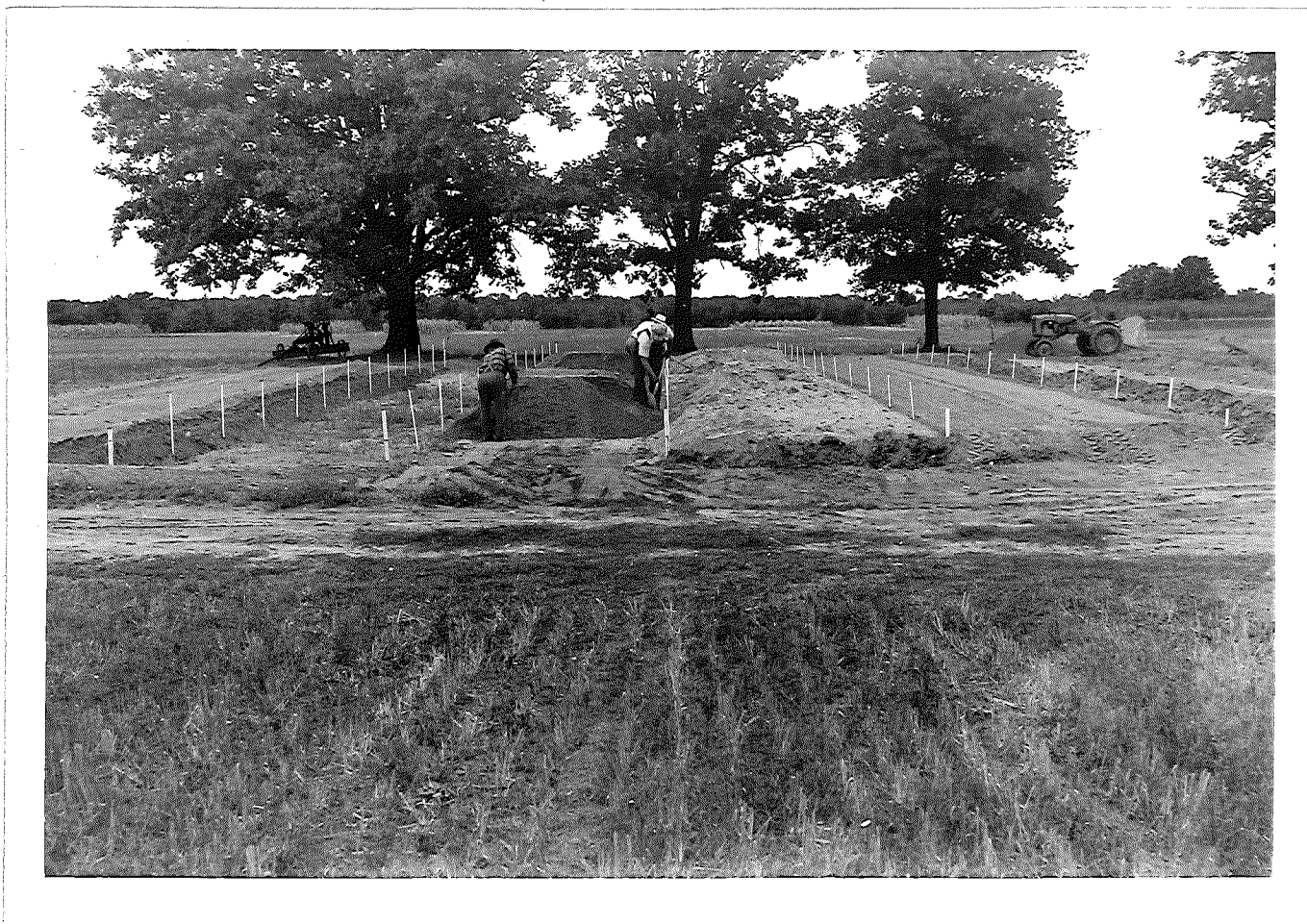
Figure 2. General view of test area showing method of mixing in top soil.
