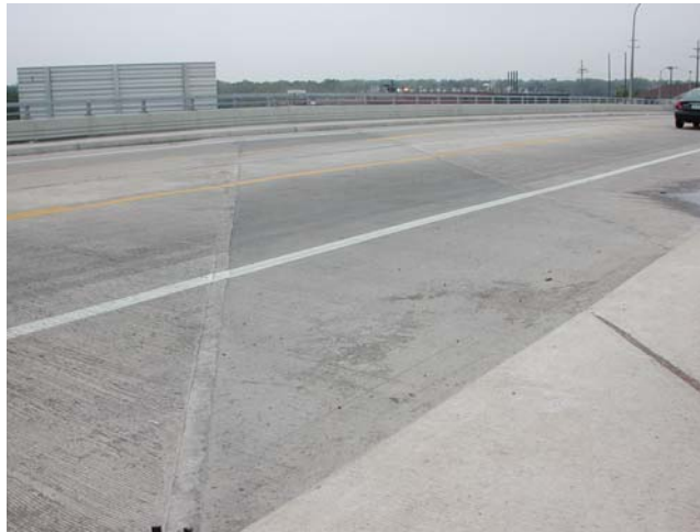
Figure 7.7: 24-month-old ECC link slab on Grove Street Bridge over I-94 (October 16, 2007)
