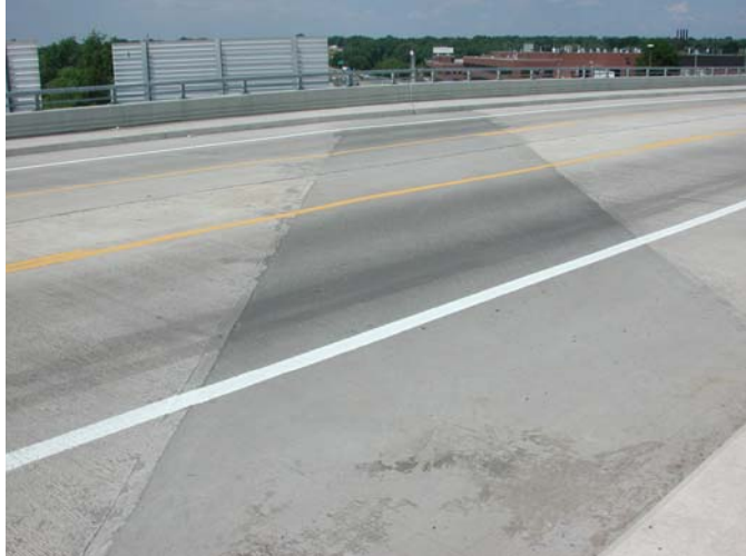
Figure 7.4: 21-month-old ECC link slab on Grove Street Bridge over I-94 (July 5, 2007)
