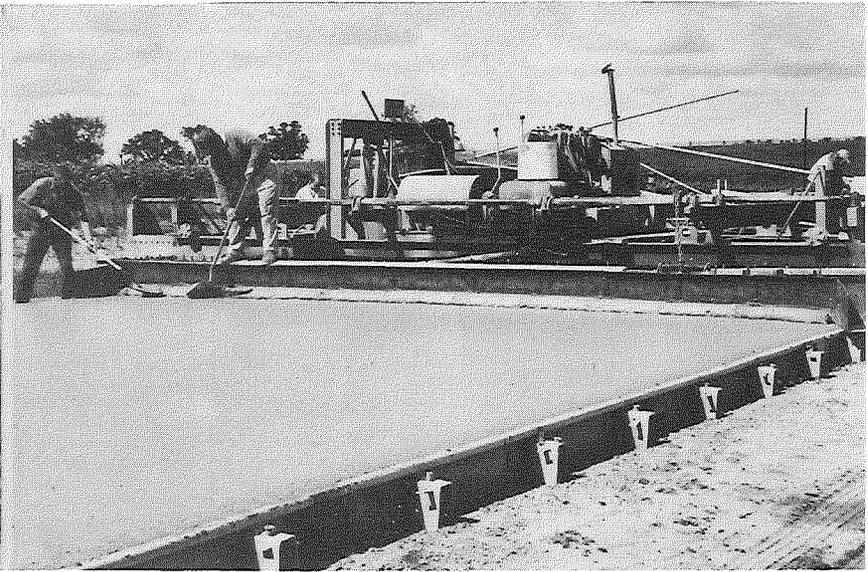
Figure 9. Final machine finishing with Heltzel Flexplane combination finisher-float machine.
