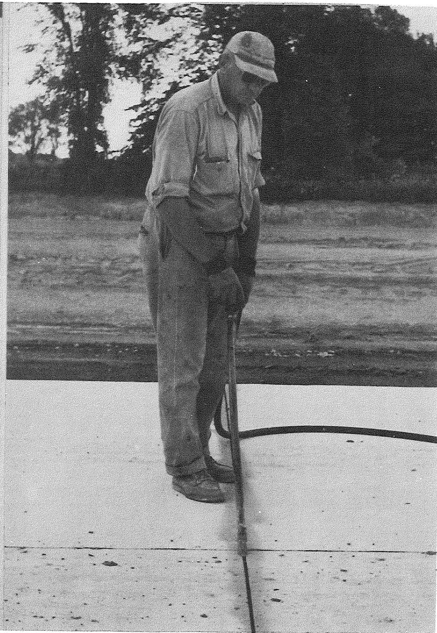
Figure 24. Cleaning joint with compressed air just before sealing.
