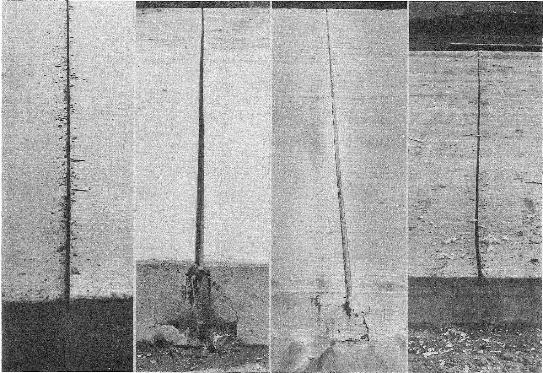
Figure 22. Typical joints before sandblasting: from left, Unitube, sawed with filler strip, sawed without filler strip, and styrofoam.
