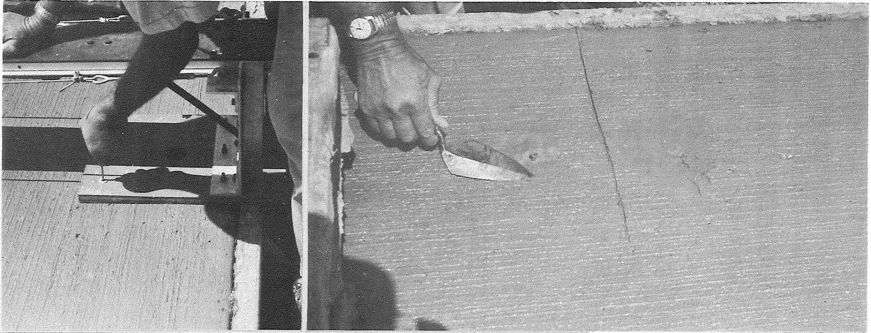
Figure 28. Setting plugs for measurement of relative joint displacement (upper left).
