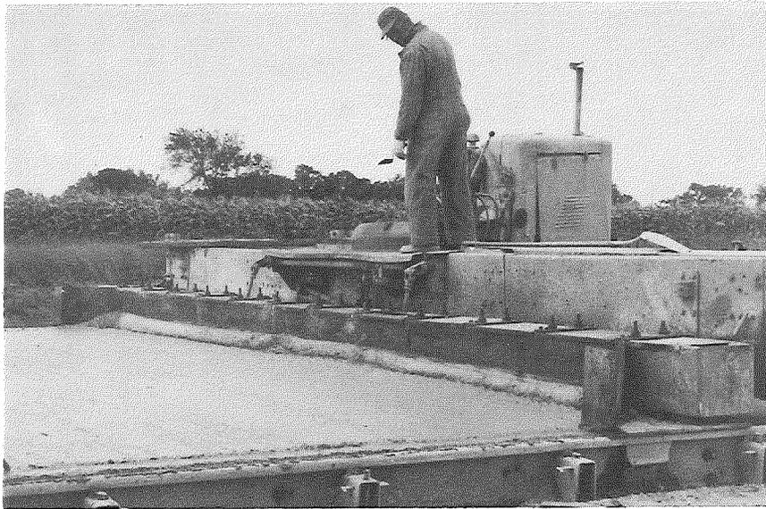
Figure 8. Initial finishing of concrete surface with Jaeger-Lakewood finishing machine.
