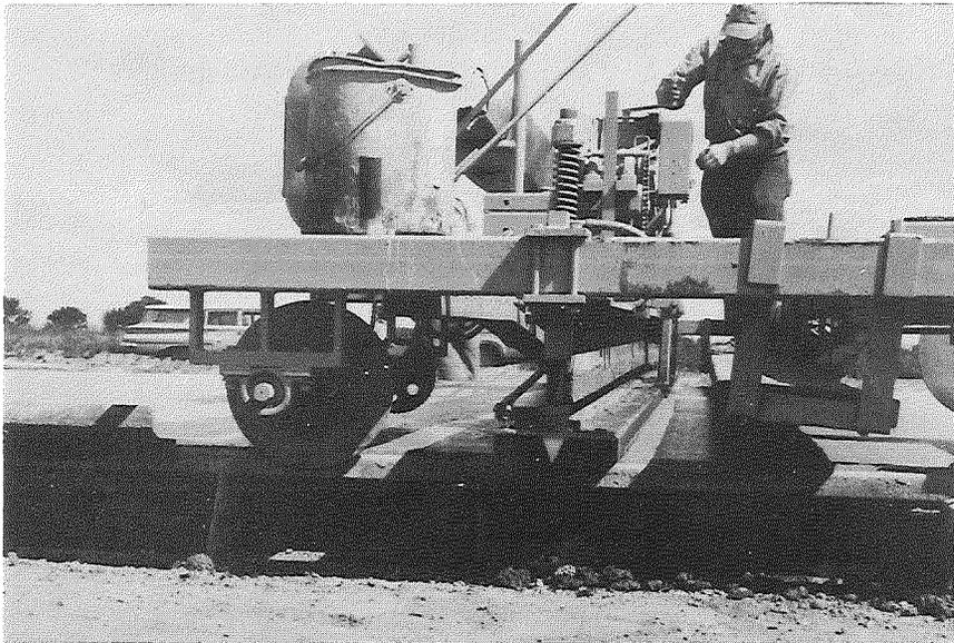
Figure 10. Unitube planter used to install Unitube, 1/4 by 2 in. premolded filler strips, and for vibrating at the locations of sawcut to form plane-of-weakness.
