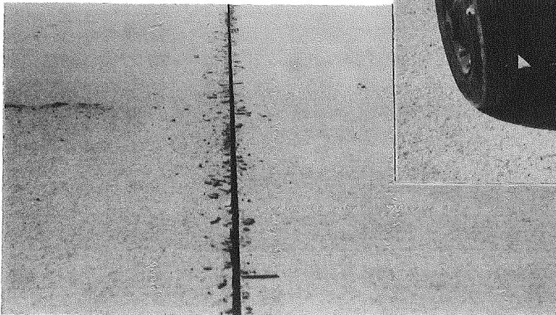
Figure 19. Condition of newly crimped joint.
