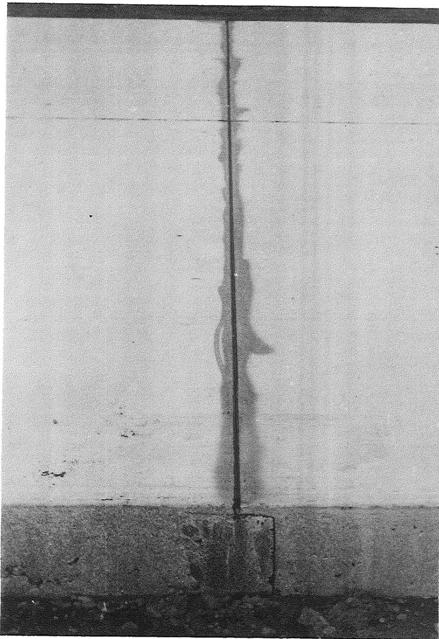
Figure 23. Condition of typical joint after sandblasting.
