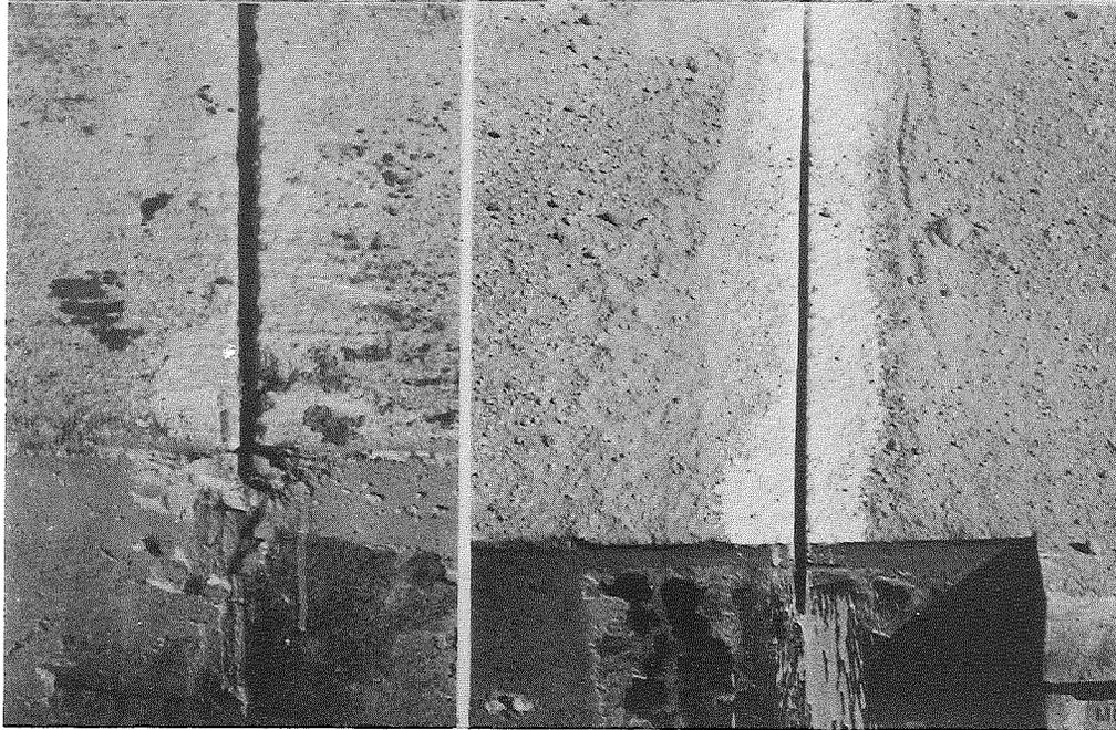
Figure 21. Sawcutting transverse joint grooves with carborundum blades is shown above. Typical plane-of-weakness cuts include one at a vibrated joint 6 to 7 hr after pour (lower left) and one at a vibrated joint 15 to 18 hr after pour (lower right).
