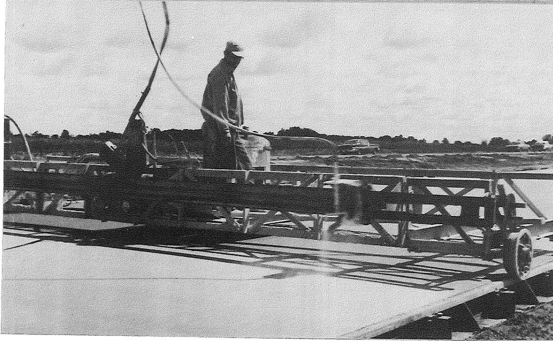
Figure 12. Final hand finishing of concrete surface (upper left).
