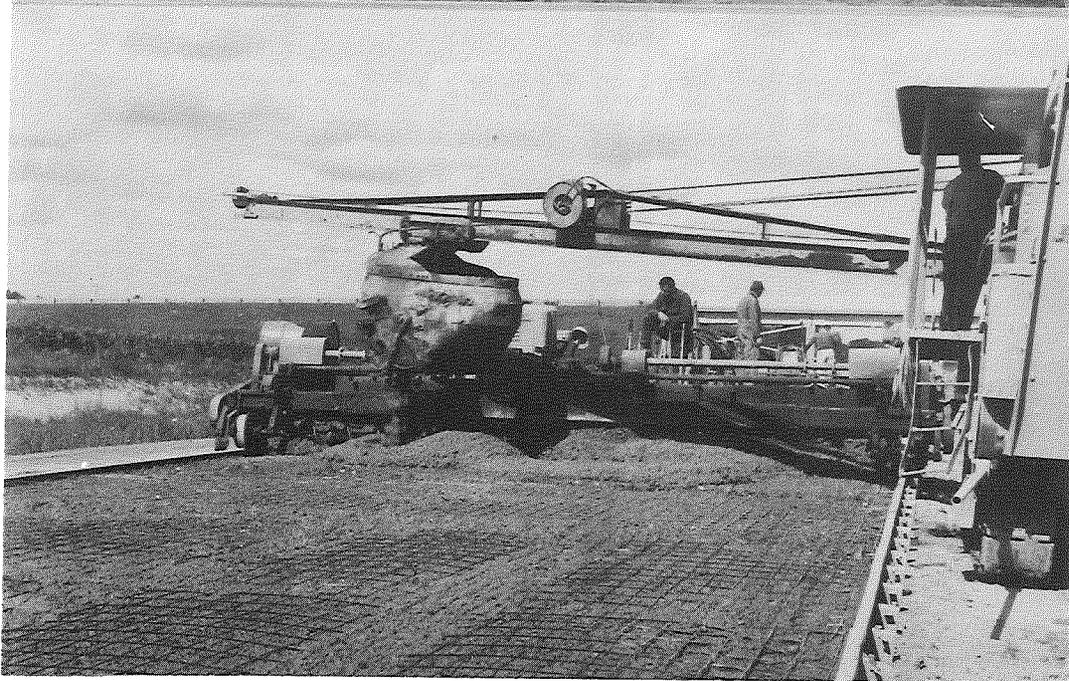
Figure 5. Placing first layer of concrete (upper left).
