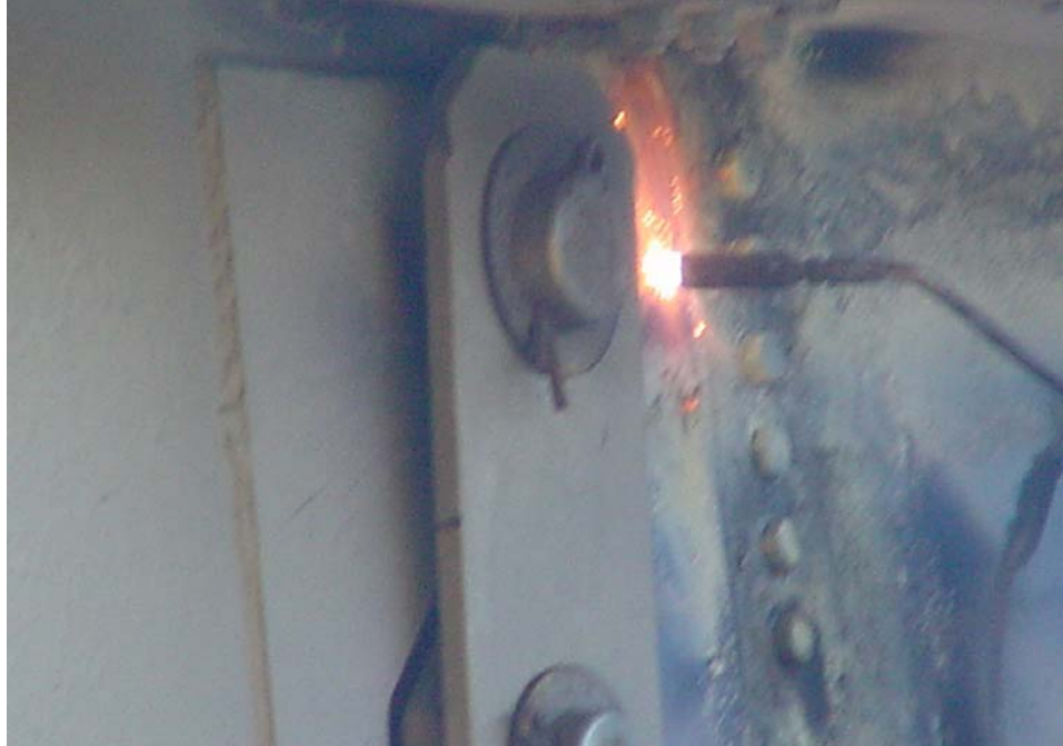
Figure 3.9 Strip heat applied close to the pin-hanger detail
