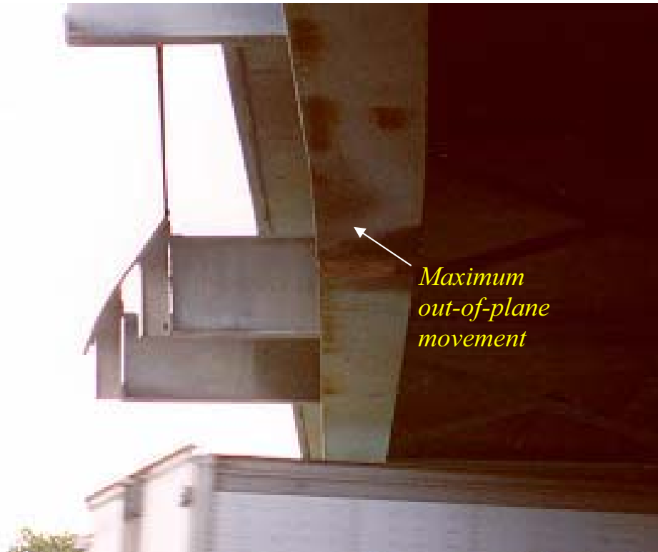
Figure 3.1 Out-of-plane movement of the Lake Lansing Road Bridge north fascia beam
