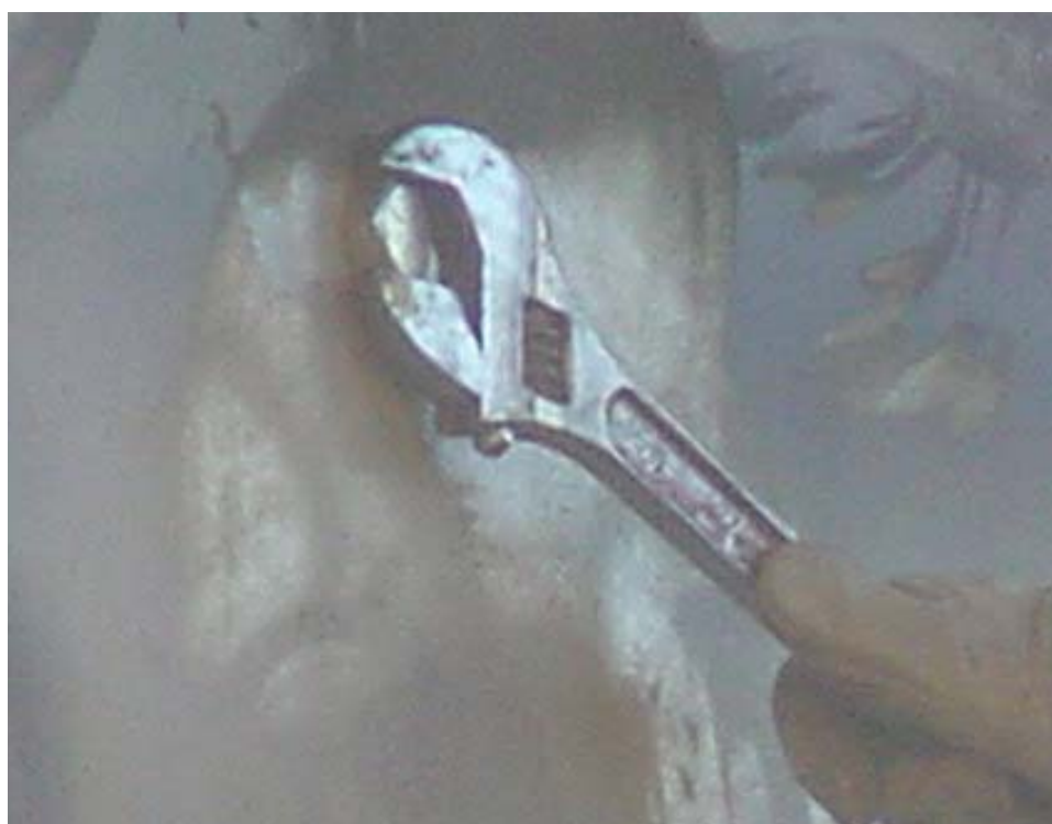
Figure 3.12 Replacement of the removed steel cores using galvanized steel bolts
