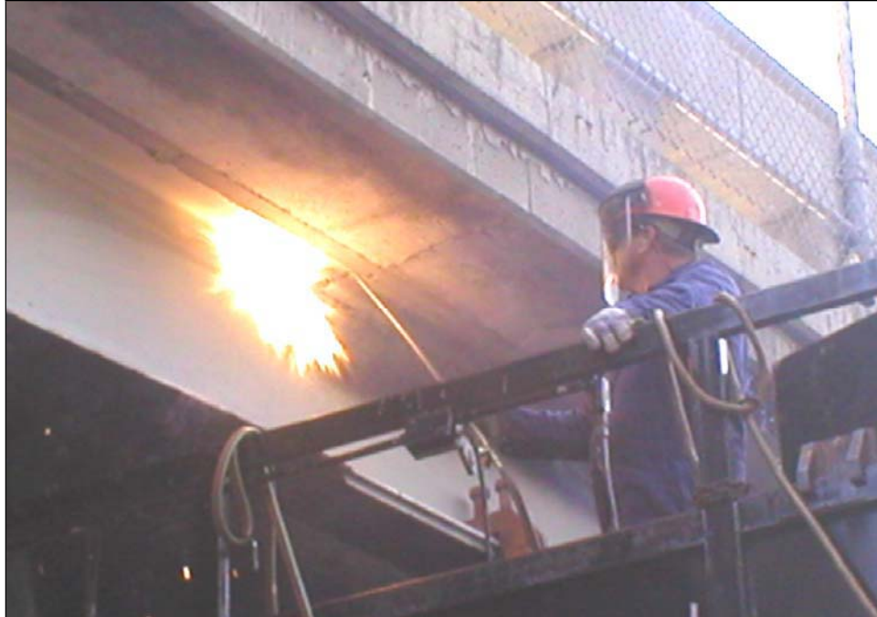
Figure 3.5 Photograph of the strip heat applied to the web
