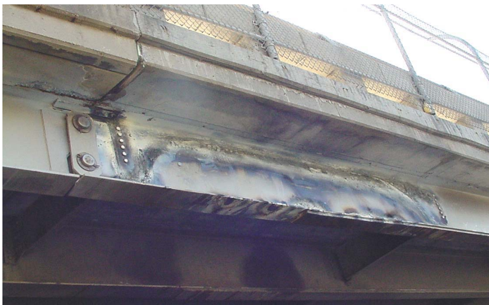
Figure 3.11 Condition of bridge girder after heat straightening repair procedure
