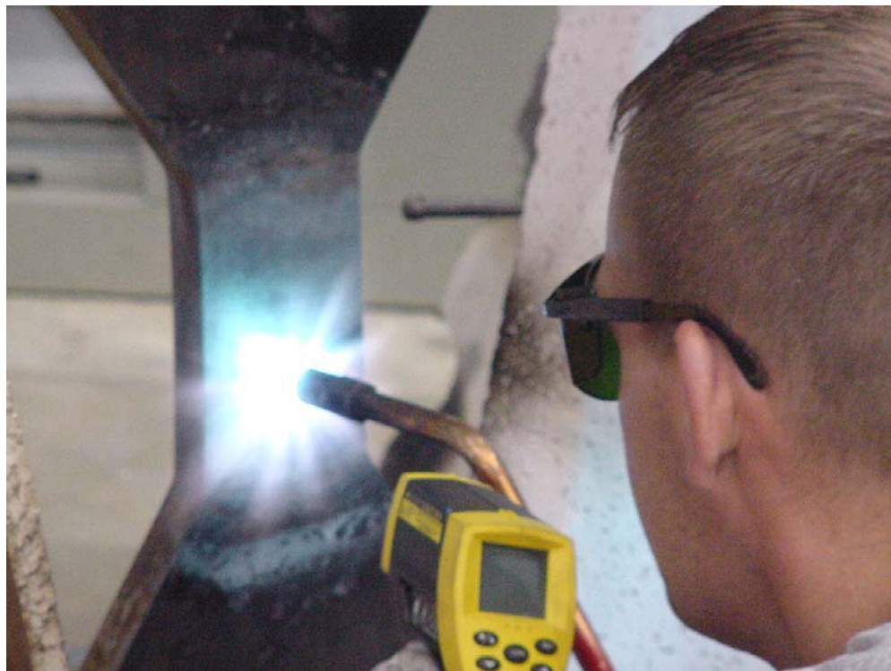
Figure 4.32 Application of the strip heat to the test area
