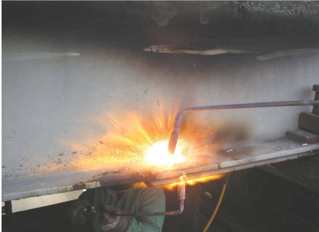
Figure 3.7 Vee-heat of the bottom flange and cover plate using two torches
