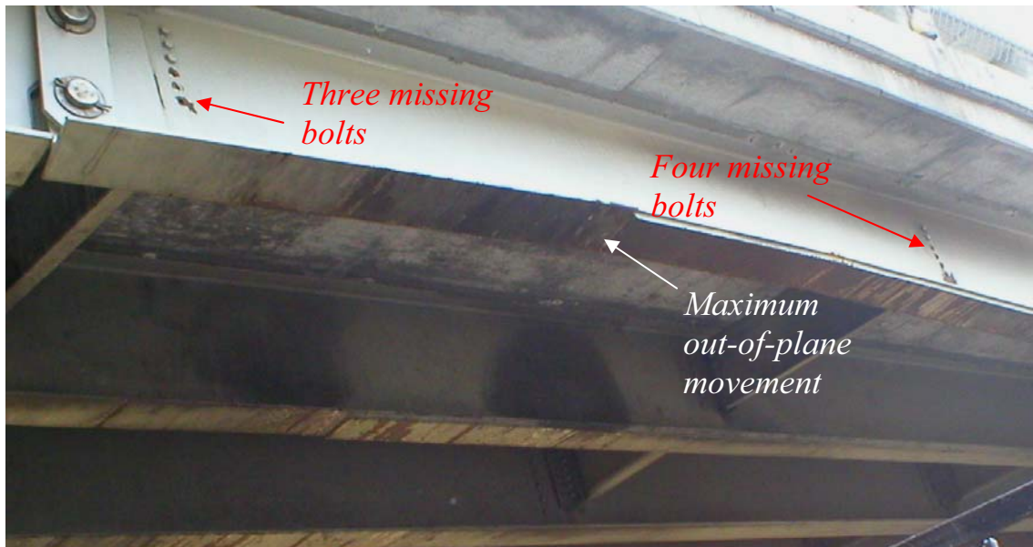
Figure 3.2 Damage on the south side of the Lansing Road Bridge west fascia beam
