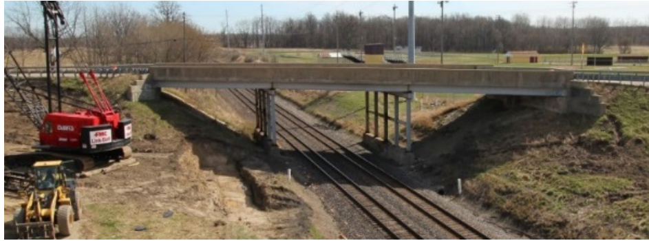
(a) Existing bridge
