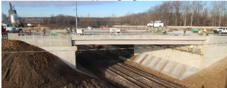
(a) Replacement bridge
