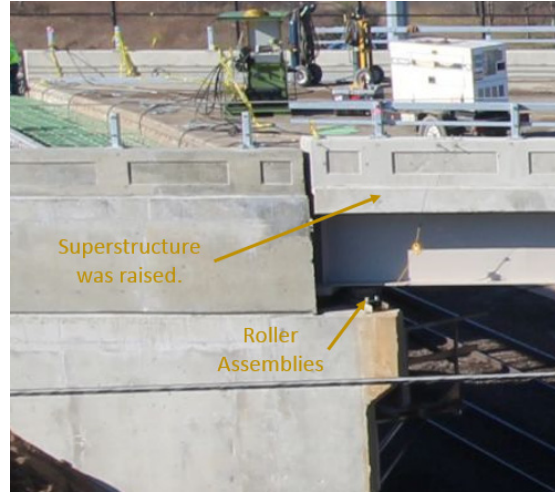
(b) Superstructure was slightly raised to remove rollers
