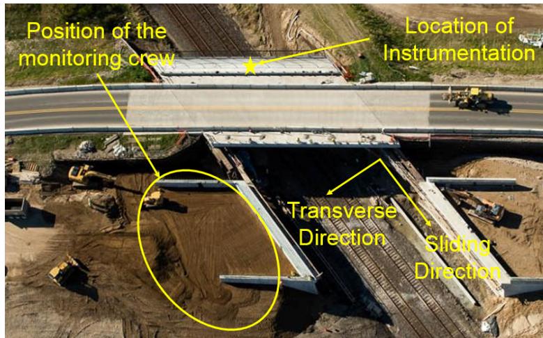
Figure 5-18. Site layout and position of sensors and monitoring crew
