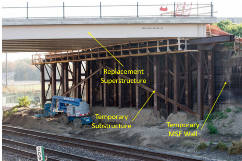
Figure 5-5. New superstructure at temporary location
