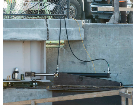
(b) Hydraulic cylinder with pulling and pushing capabilities
