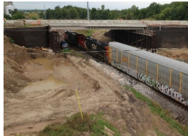
(b) During the construction of replacement substructure
