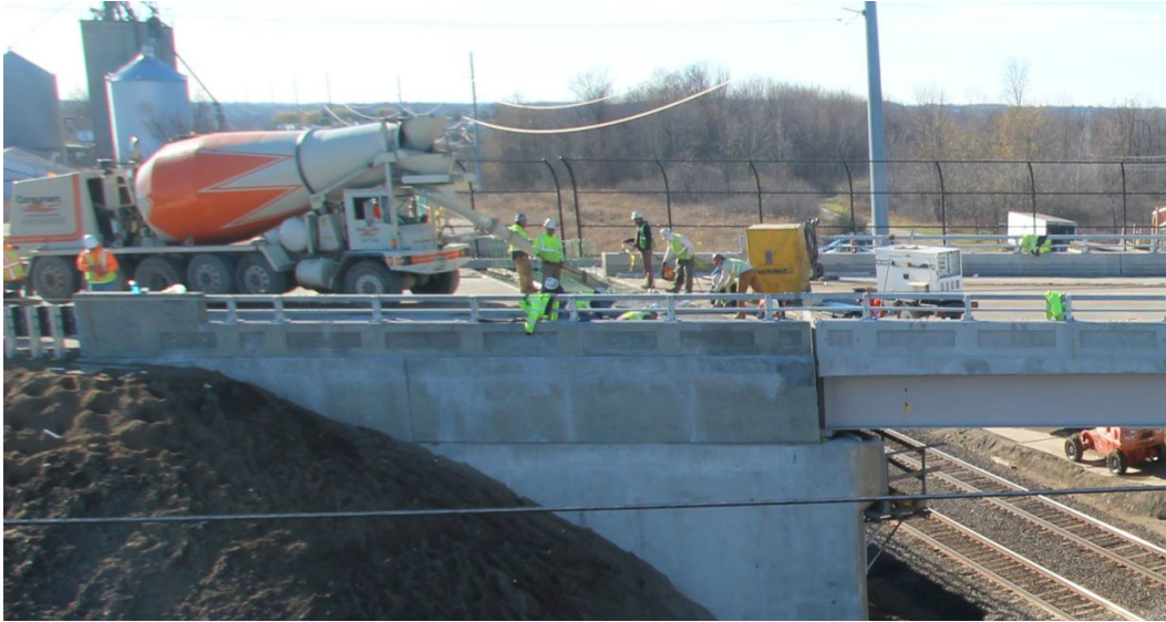
Figure 5-13. Placement of approach slab
