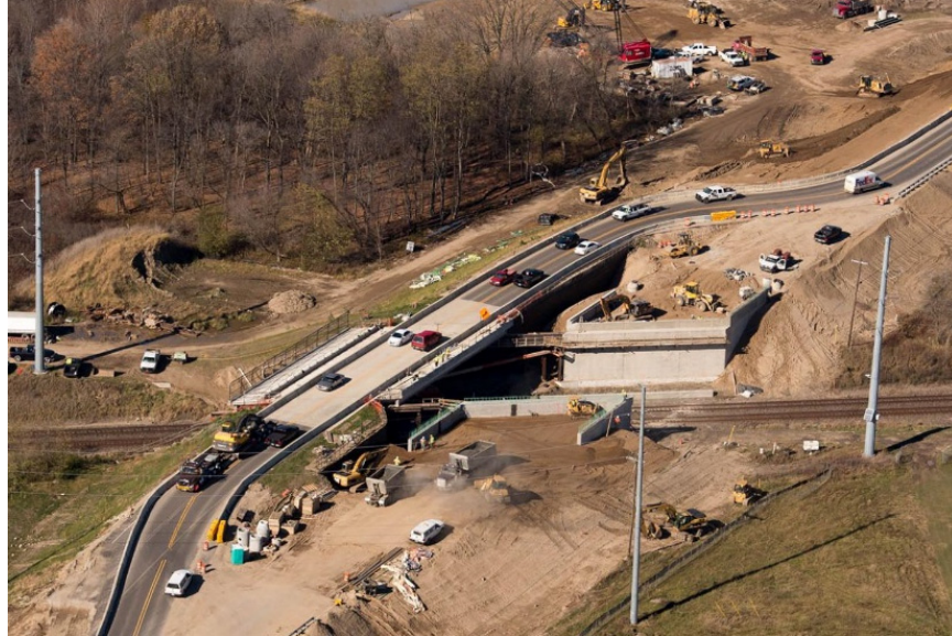
Figure 5-7. Replacement superstructure as the temporary runaround for traffic
