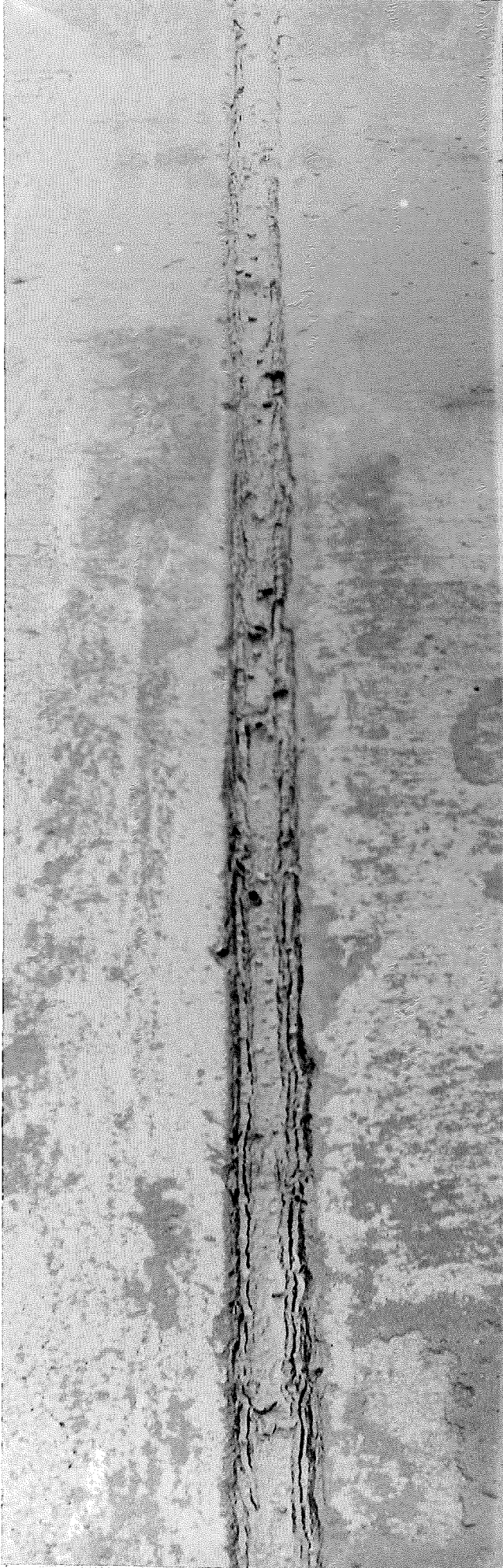
Material A, Station 288+63 No failure.
