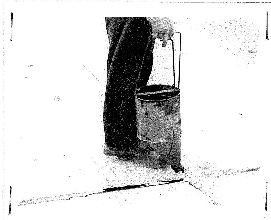
Figure 7. Close-up view of pouring operations.
