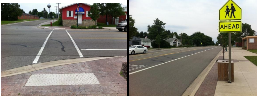
Crosswalk with warning road sign
