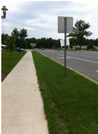
View of sidewalk facing south along M-37
