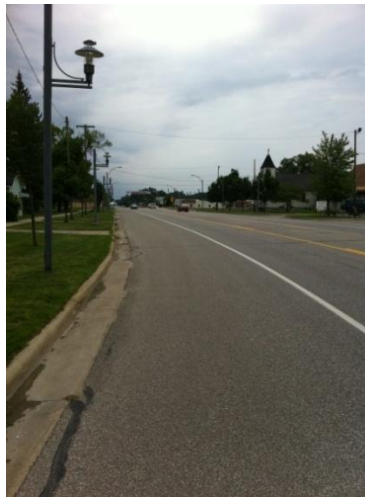
View of wide shoulder facing south
