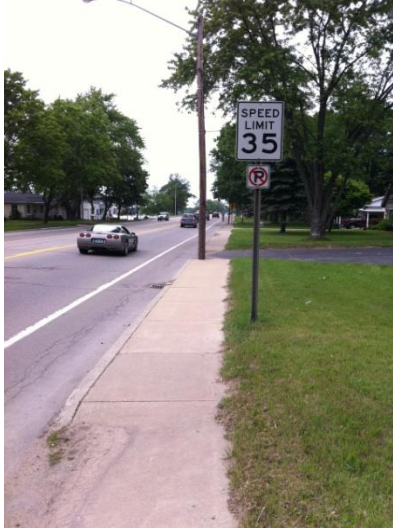
Sidewalk directly adjacent to pavement
