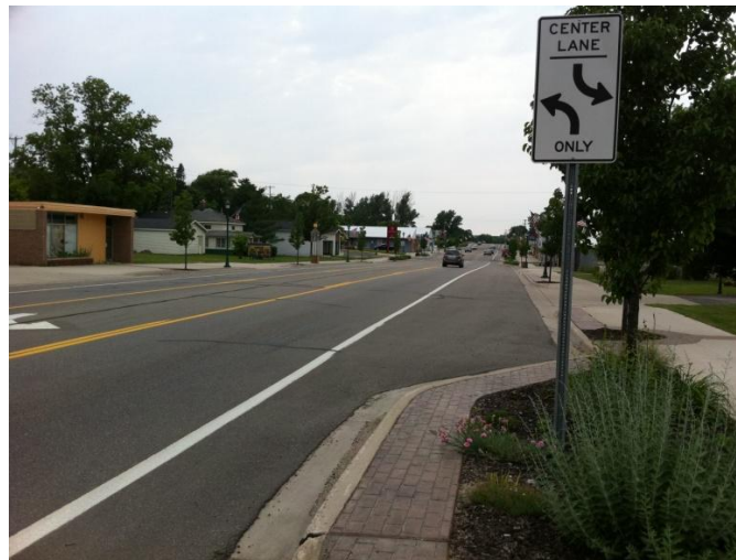
View of parking lanes facing west
