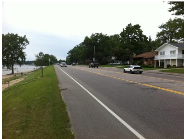
View of bike lane facing north
