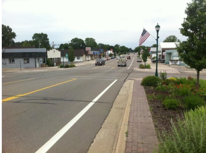
View of bike lanes facing west
