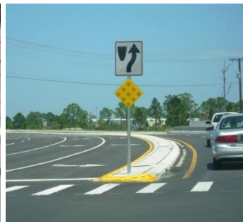
Knockdowns of signs in the median may be avoided with use of an object marker.
