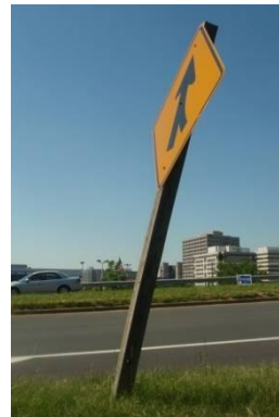
Visibility of sign will diminish if not vertically straight.
