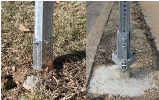
Two types of breakaway designs.
