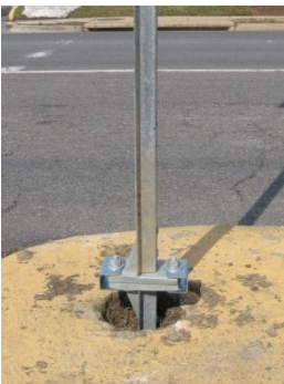
Breakaway treatments for u-channel posts.
