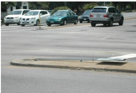
Knockdowns of signs in the median may be avoided with use of an object marker.
