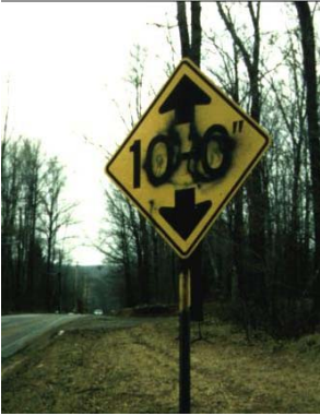
Sign damaged by overpainting.
