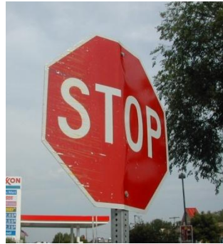
Bent signs can be repaired in the field
