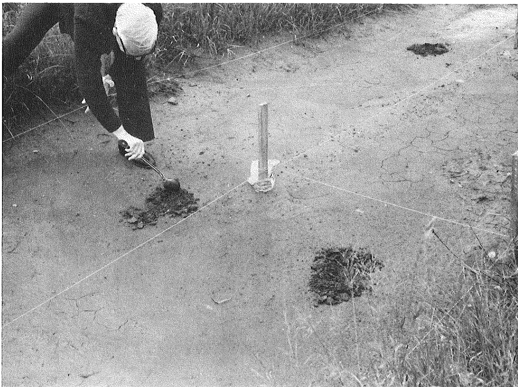
Figure 8. Showing lack of bonding of the test areas.
