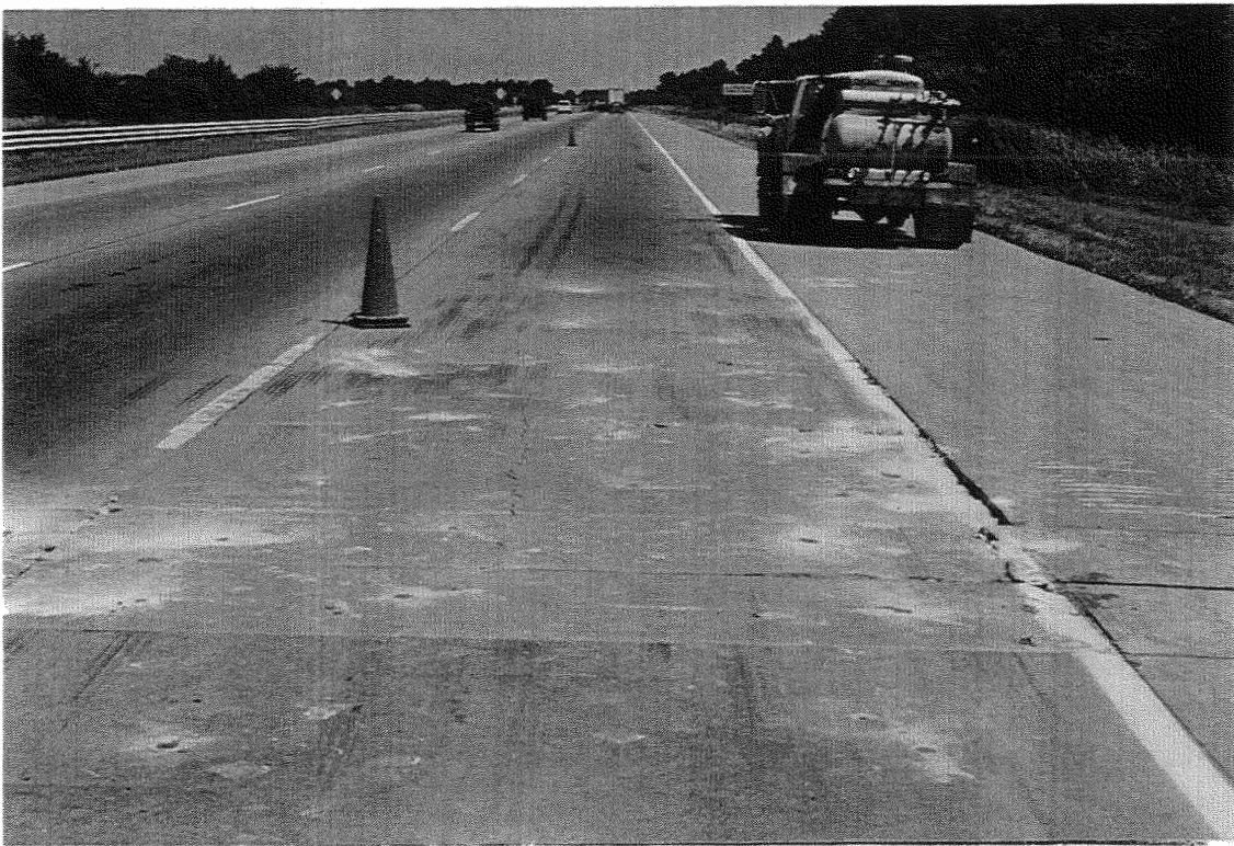
Figure 8. Raised slab after treatment.
