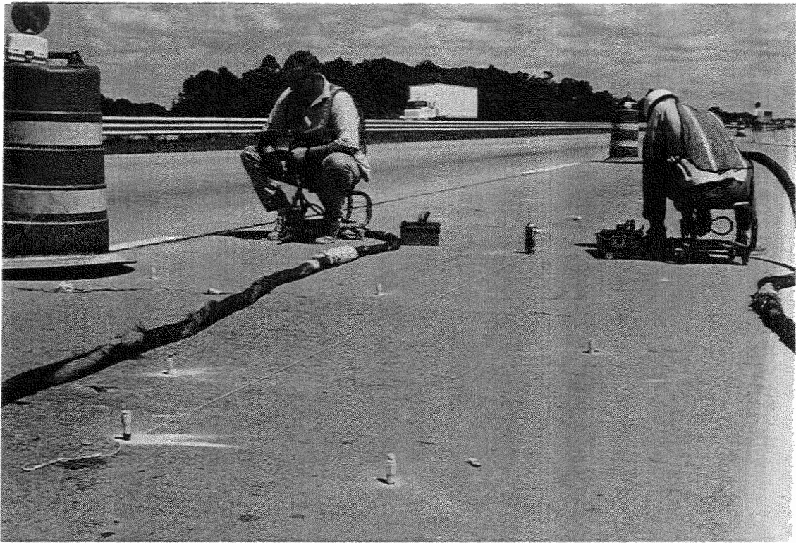
Figure 3. Injecting material through pavement.
