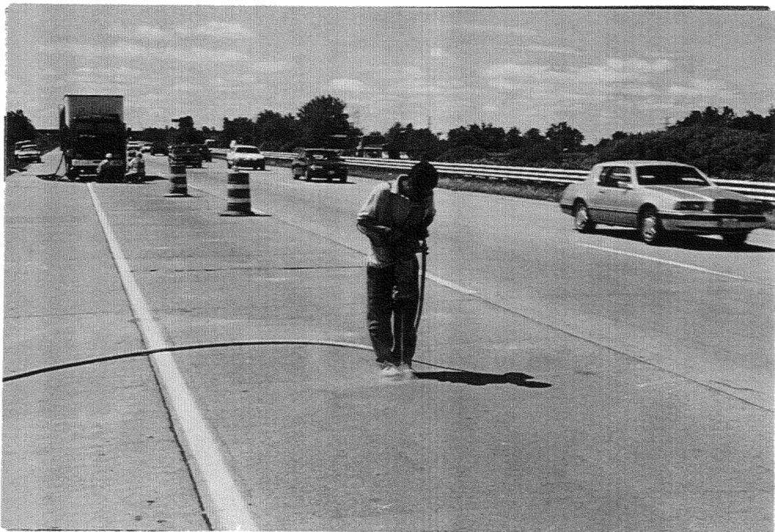
Figure 2. Drilling holes in concrete pavement.
