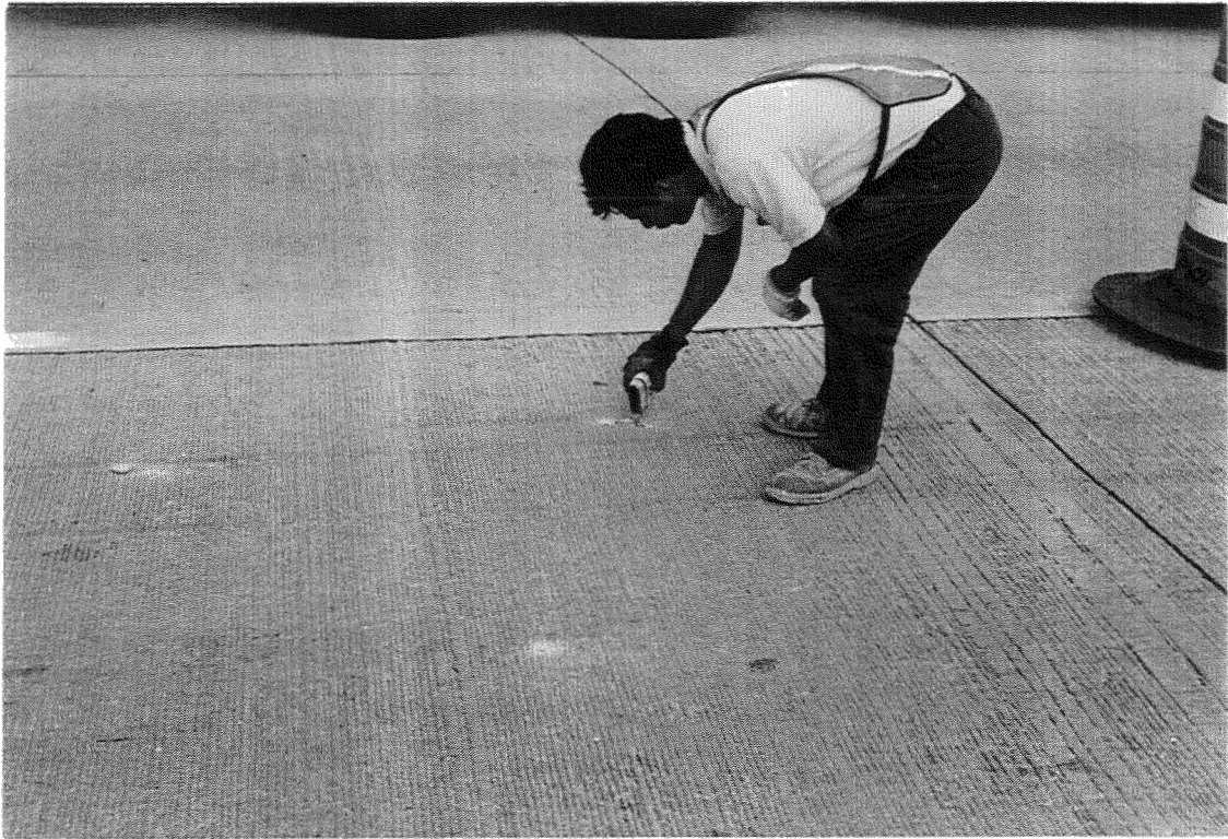
Figure 9. Grouting the drilled holes.
