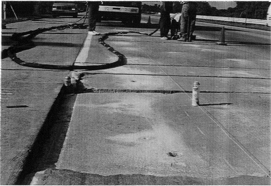
Figure 7. Four-inch settlement before treatment.
