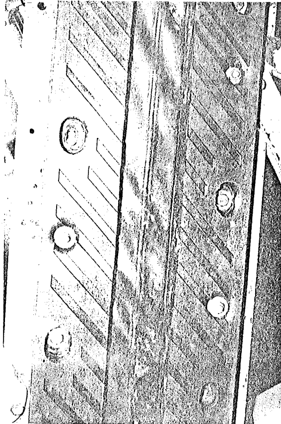
Figure 4. Fel-Span CS 3-in. system in extension at a 60-degree angle of crossing. Sealing gland is stretched taut.
