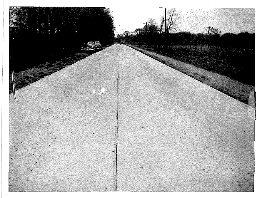
A. General view looking north showing general condition of pavement.
