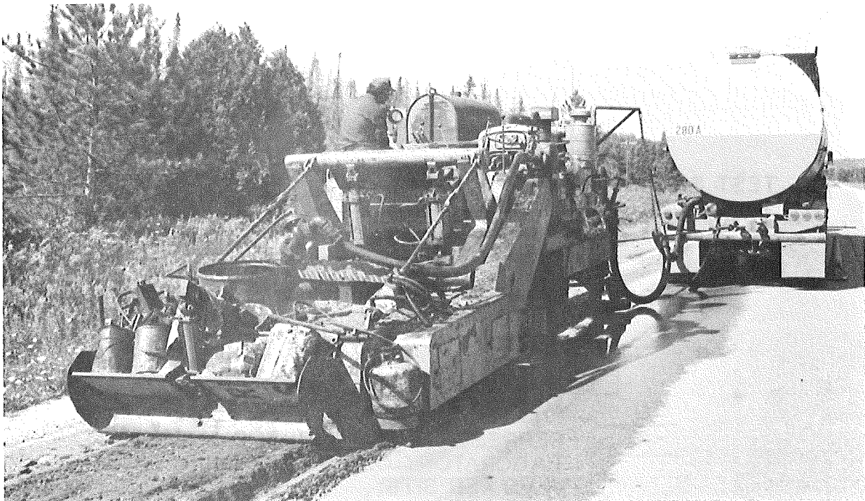
Stabilization of shoulders along US 131 in Charlevoix County, single-pass stabilizer adding and mixing foamed asphalt following asphalt tanker.
