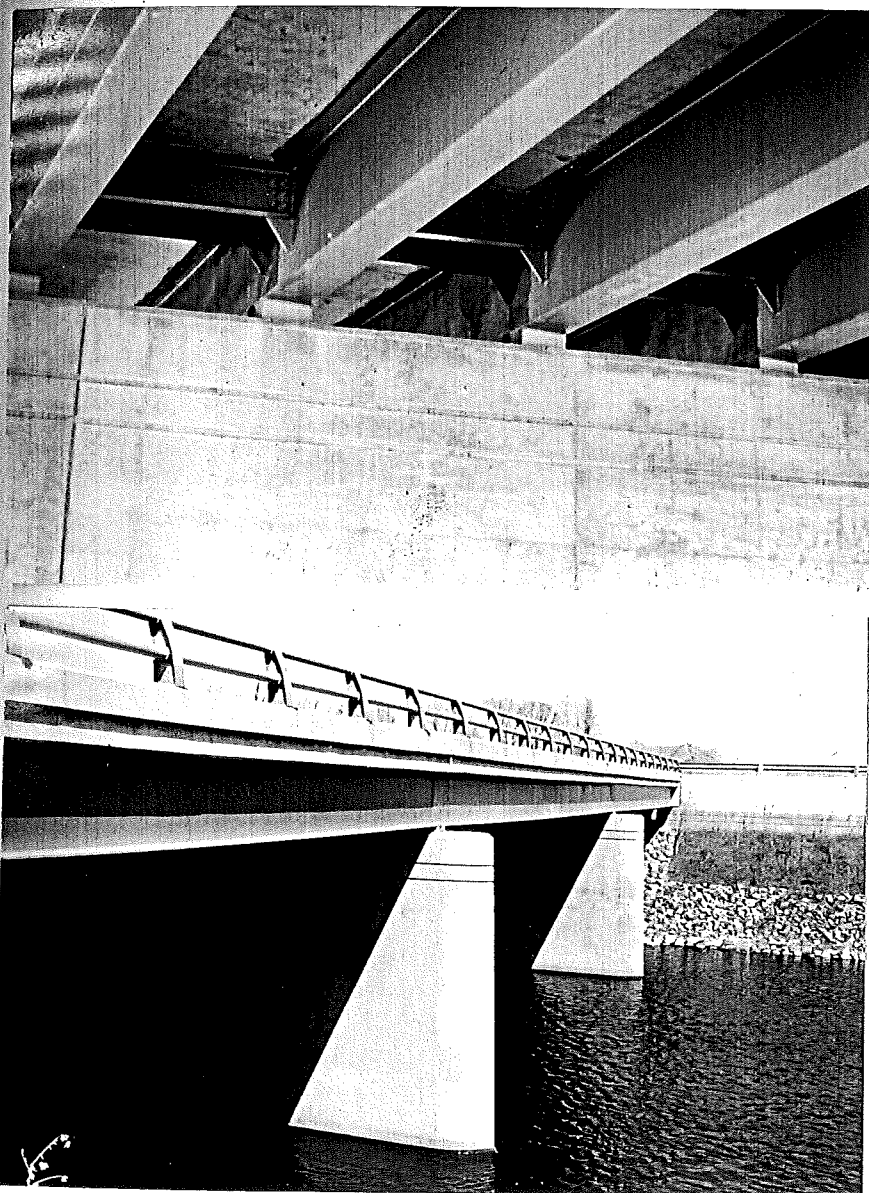
Figure 3. Good condition of test coatings on most steel after 3-1/4 years of service on westbound Shiawassee River bridge.
