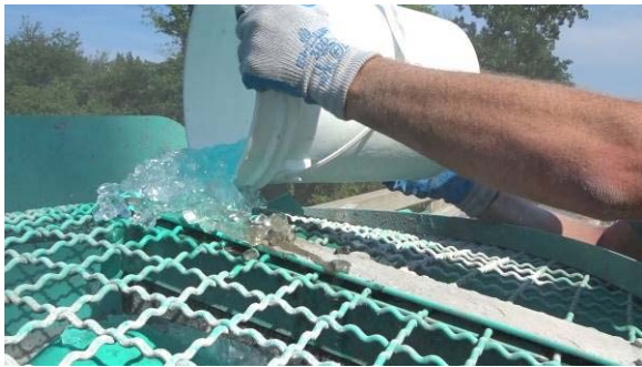
(c) Addition of liquid with cubed ice
