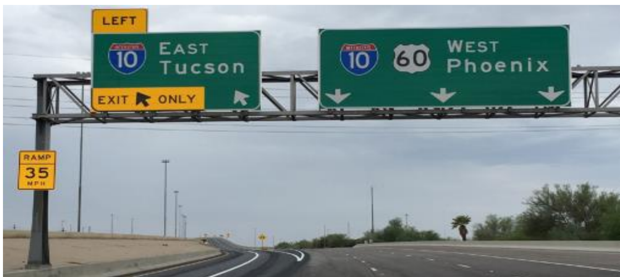
Figure 4. Improved US-60 and I-10 Interchange in Tempe, Arizona [20]
