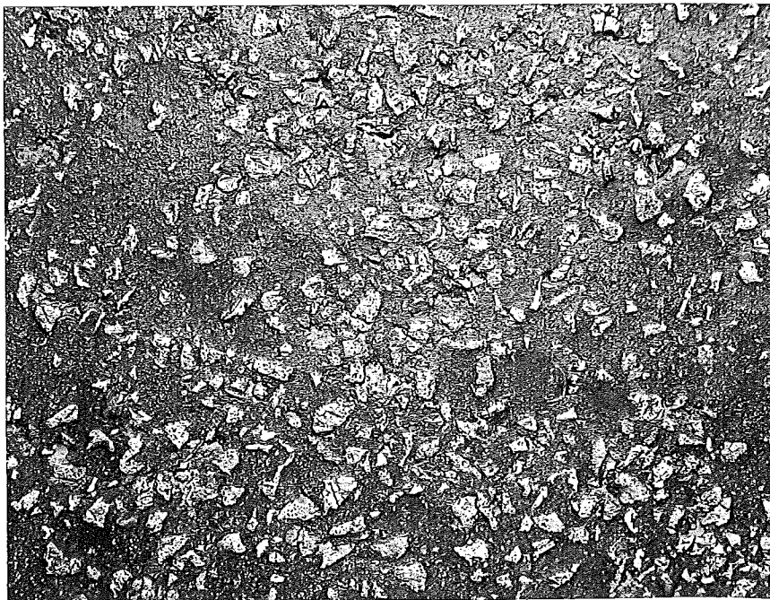
B. View of surface showing typical condition of aggregate.
