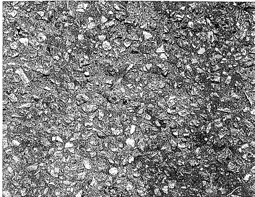
B. View showing typical condition of aggregate.
