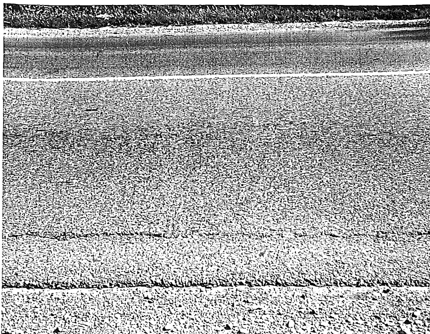
A. Typical condition of surface. Slight pitting.
