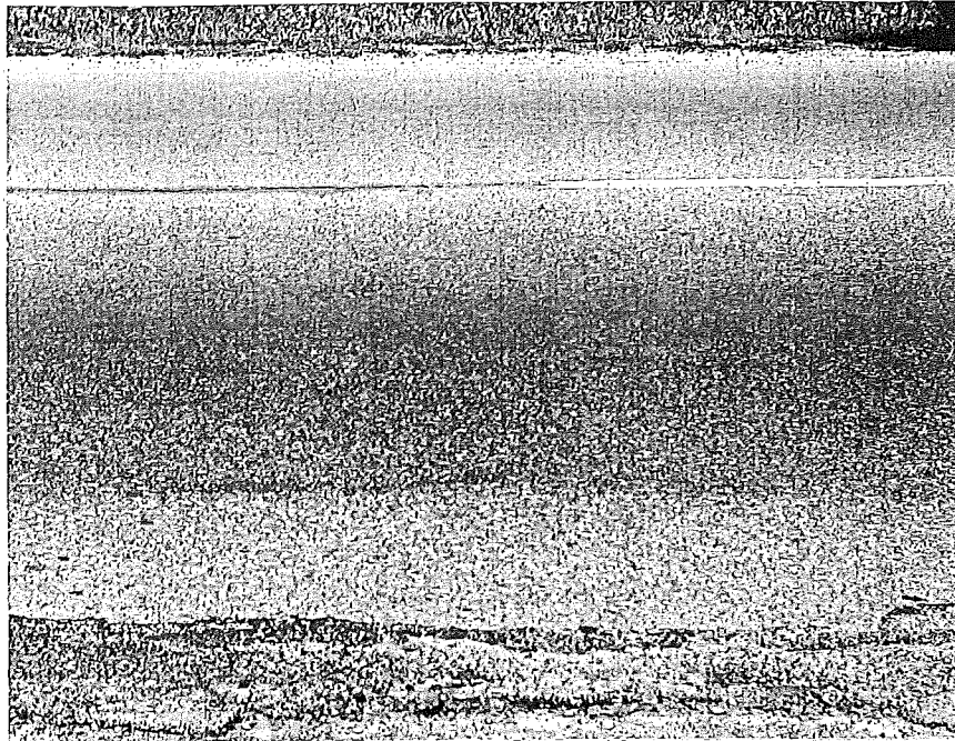
A. Typical condition of surface. No pitting.
