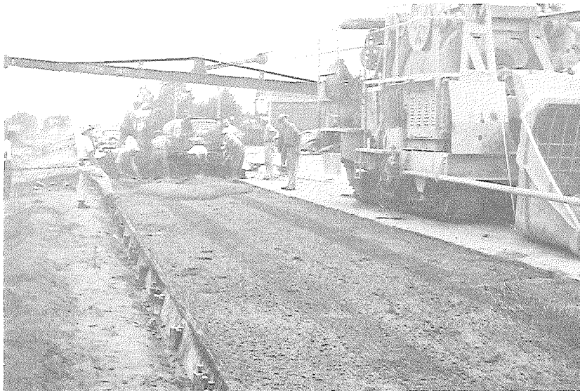
IN CONCRETE ROADWAY
