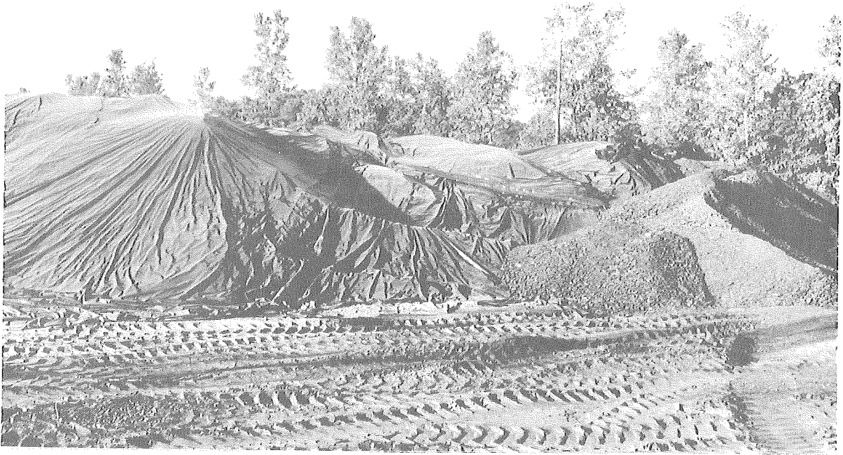
Figure 1. Covered stockpile of reclaimed pavement material.
