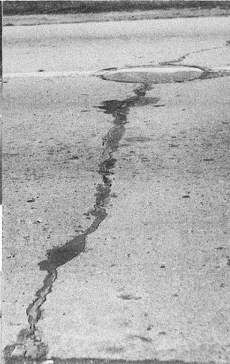
▲ Station 13+98. Transverse cracks developed over sanitary sewer pipes.
