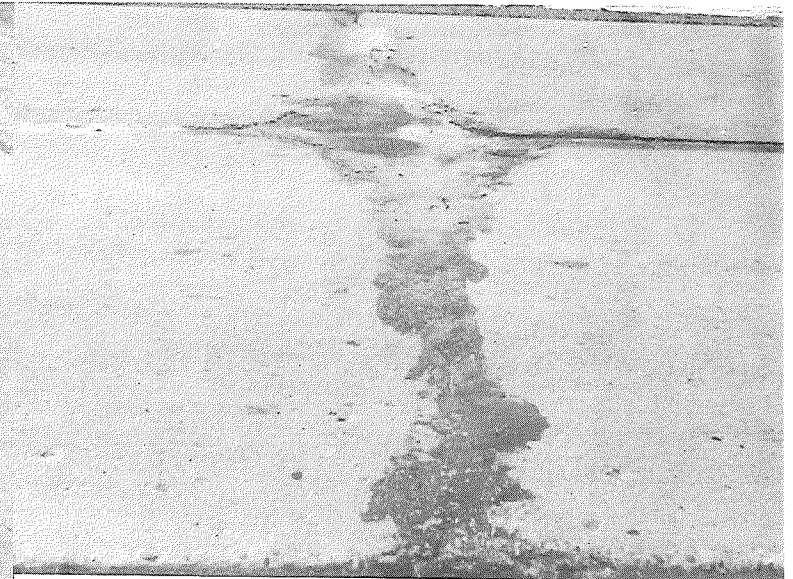
▲ Station 469. This joint subject to pumping, showed disintegration typical on Contract 5, with heavy spalling and corner breakage.
