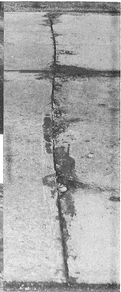
▲ Station 278+20. This patch, placed in 1954 by part-width construction, was subject to pumping along its transverse, center, and shoulder edges; note differential slab elevation at centerline.
