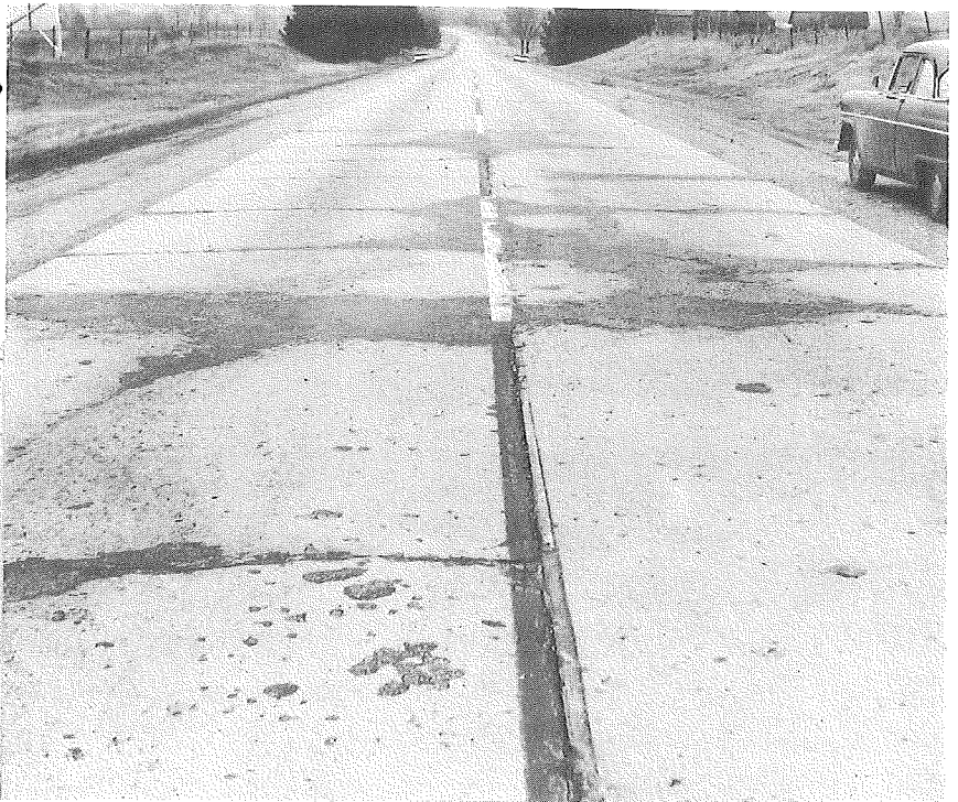
Station 89+49. The condition of this expansion joint was typical of those in Contract 3; note longitudinal cracking (top). occasionally found in this project.
