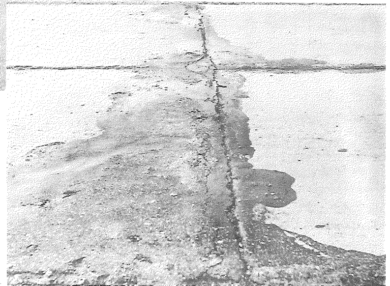
▲ Station 469. This joint subject to pumping, showed disintegration typical on Contract 5, with heavy spalling and corner breakage.
