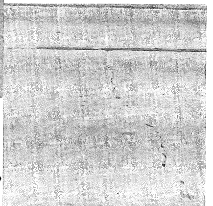
▲ Station 13+98. Transverse cracks developed over sanitary sewer pipes.
