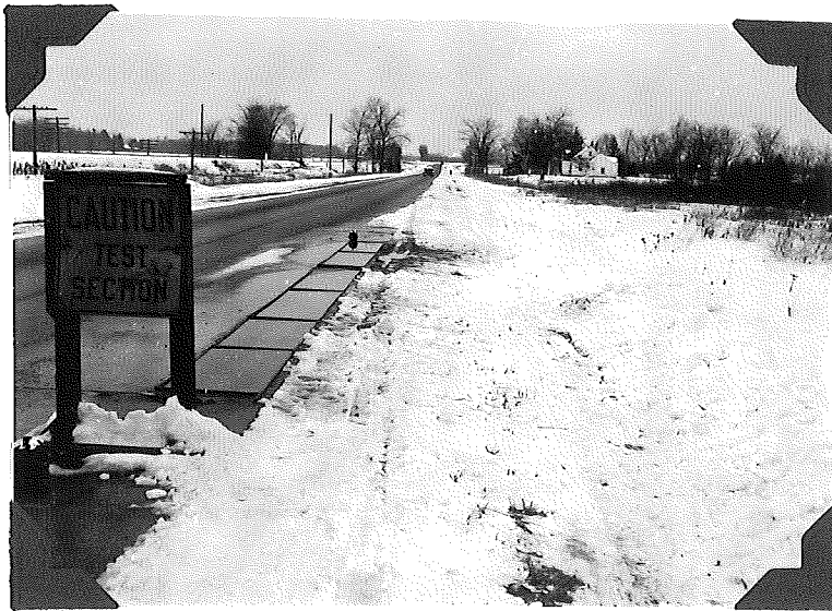
Figure 1. Typical installation of test panels.
