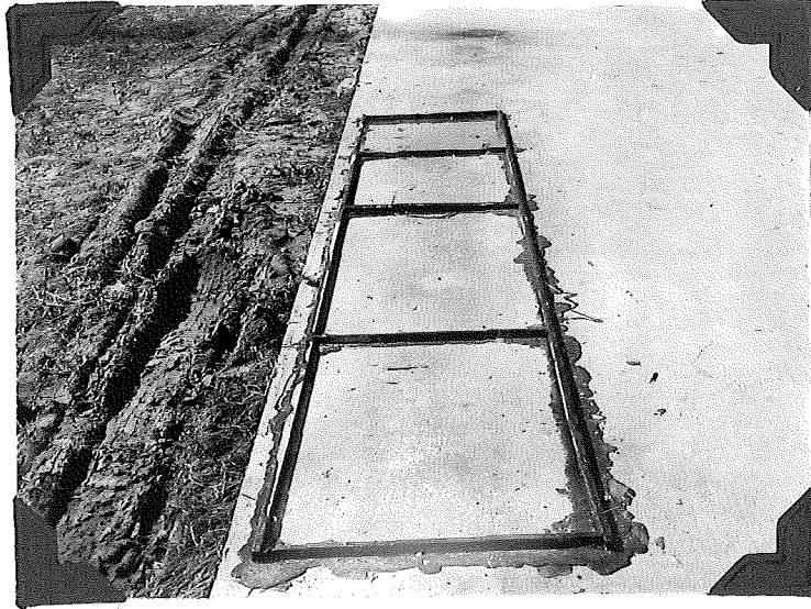
Figure 3A. Calcium Chloride panel of test area No. 1 after 26 cycles. Pavement 4 years old containing Orvus. Project 18-20,C3. Station 463+50. No scale.
