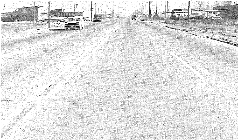
Method 3: AE-3 and sand separation course. North from 128+00
