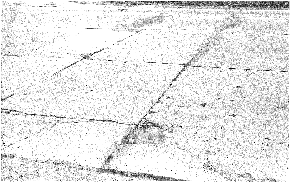
Figure 21. Repair at contraction joint in 7-1/2-in. capping with similar repair of foreground widening lane (Dec. 1959). 281+33 - Method 4.
