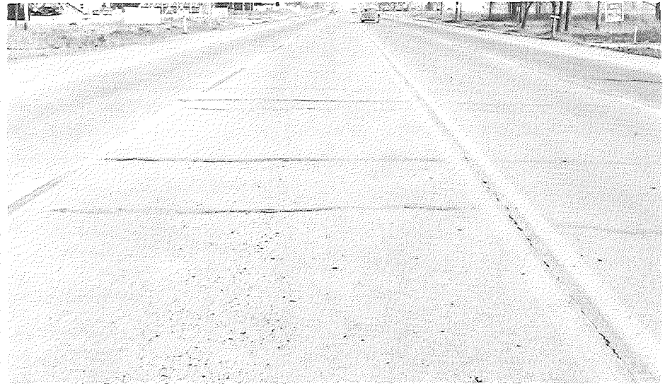
Method 2: Direct bonding, reinforcement through contraction joints. North from 346+00
