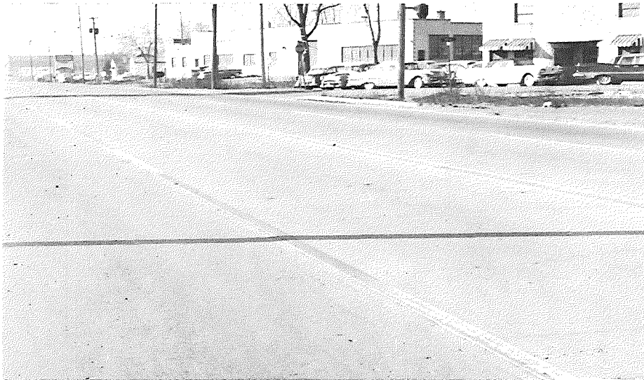
Method 1: Direct bonding, open contraction joints. North from 23+00.
