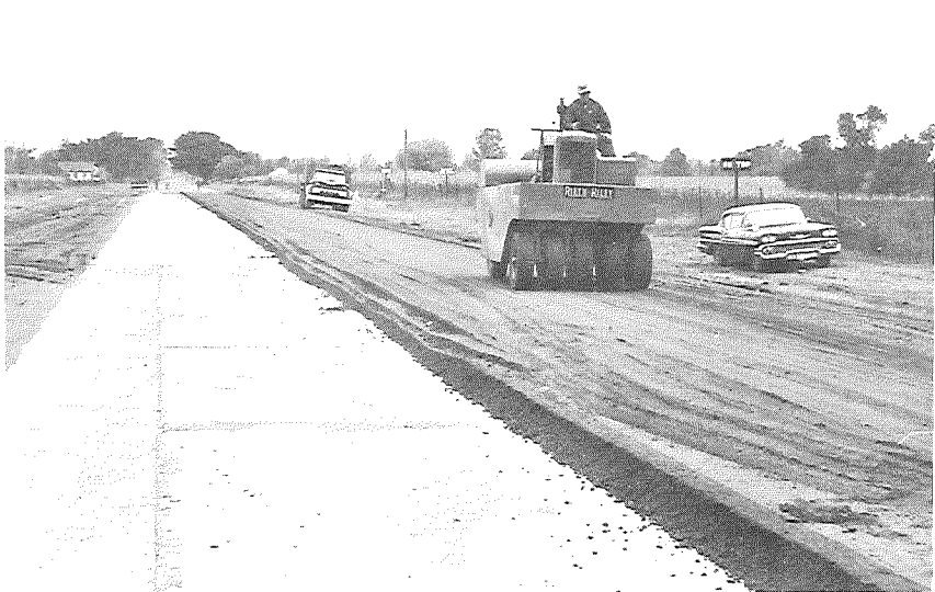
Figure 5. Construction of 23A gravel section, showing placement of gravel with asphalt paver (upper left), drying of cushion by use of windrow (upper right), compaction in progress (lower left), and appearance of completed cushion (lower right).
