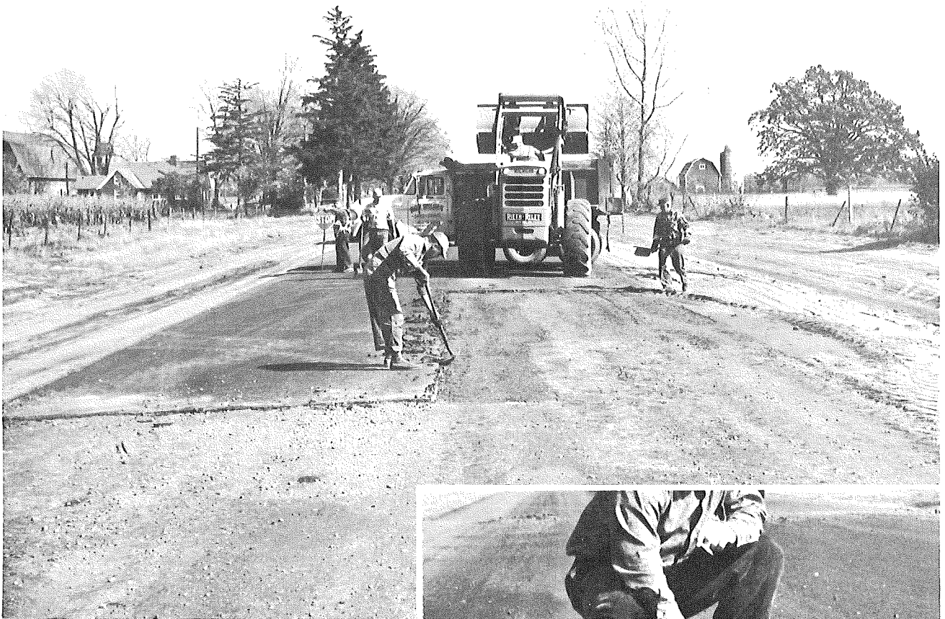
Figure 9. Removal of asphalt leveling course from distressed 23A gravel cushion (top), and appearance of cushion when exposed (center). Rutting is shown at bottom.
