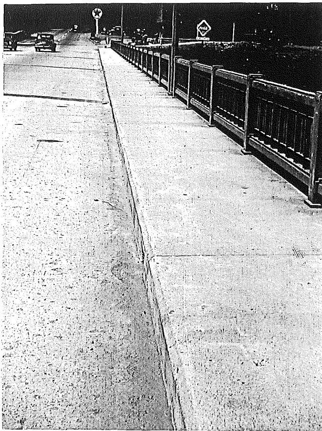
Fig. 2. East walk - no scale. Constructed with Orvus.
