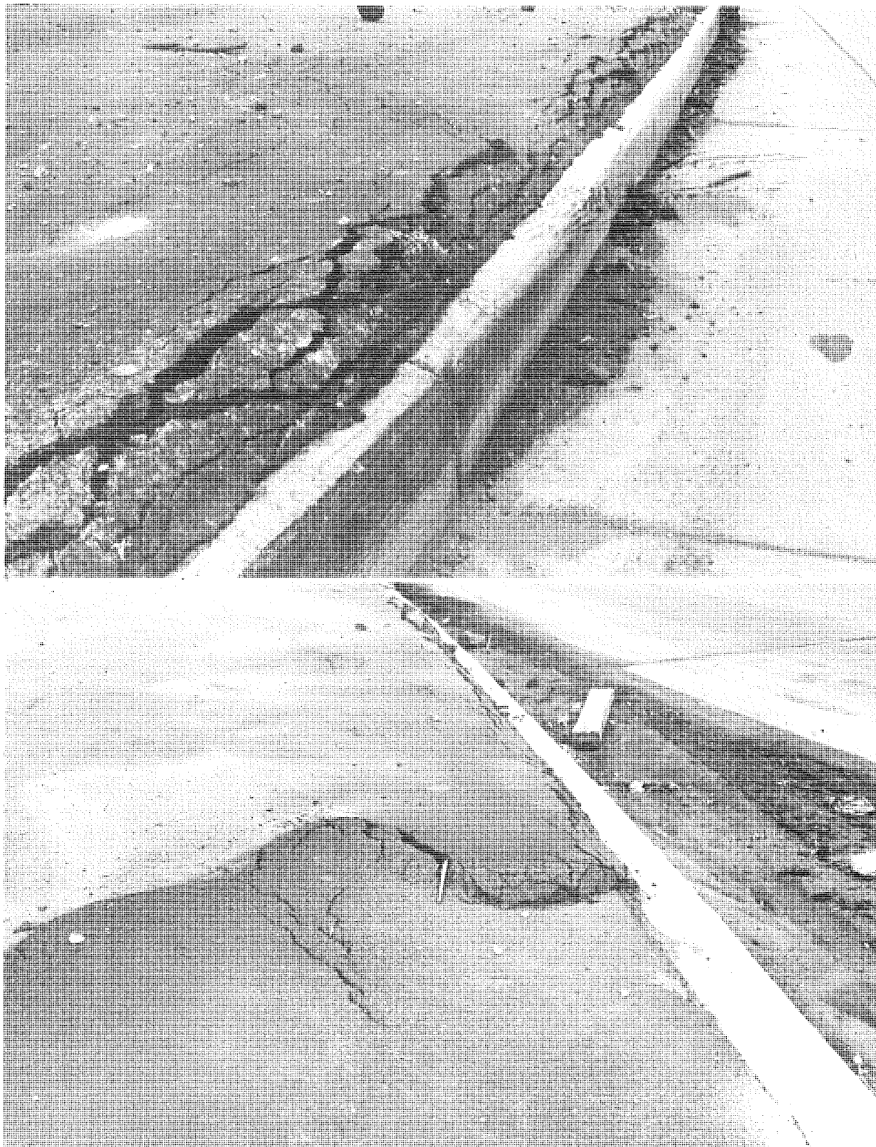
Figure 3. Bituminous surface, Dearborn St traffic island, constructed over base of steel furnace slag (1968).
