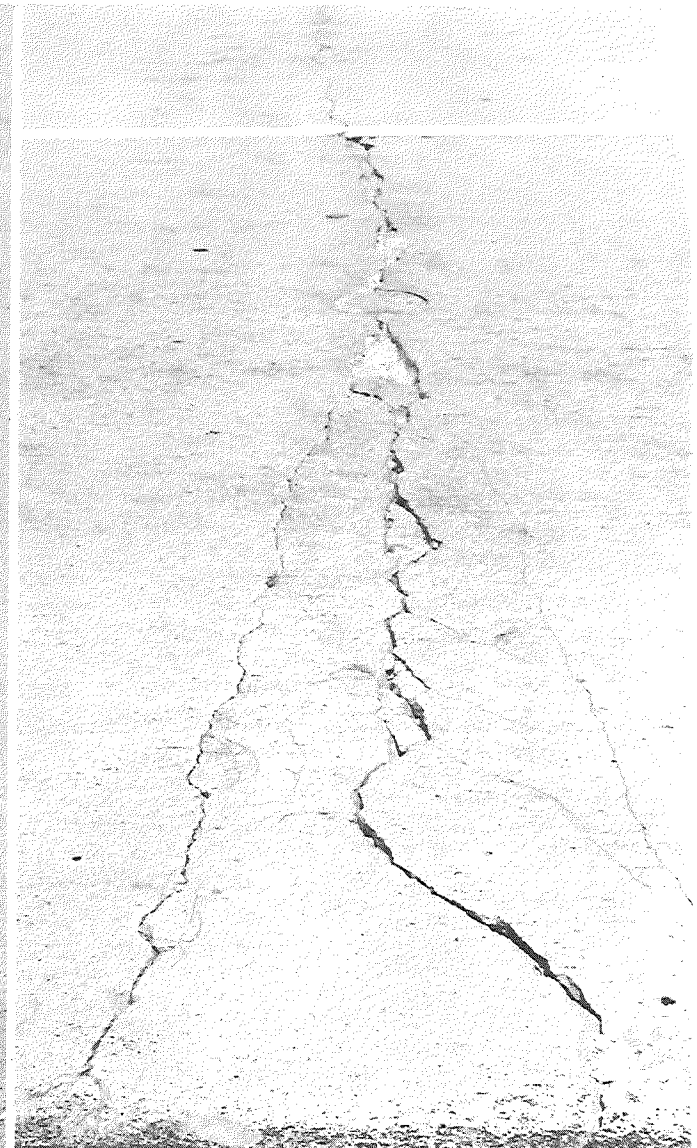
Sta 875+90, eastbound roadway (photo: April 1962)
