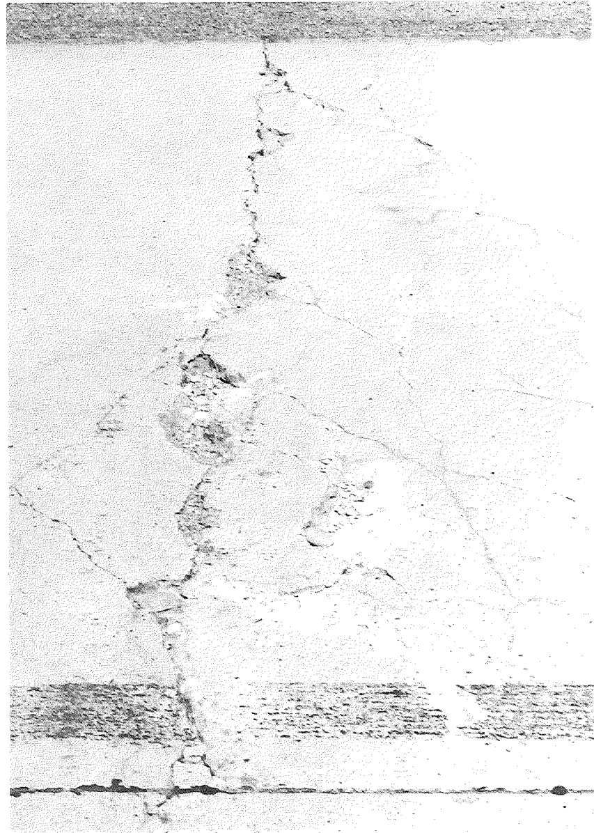
Sta 1017+03, eastbound roadway (photo: April 1960)
