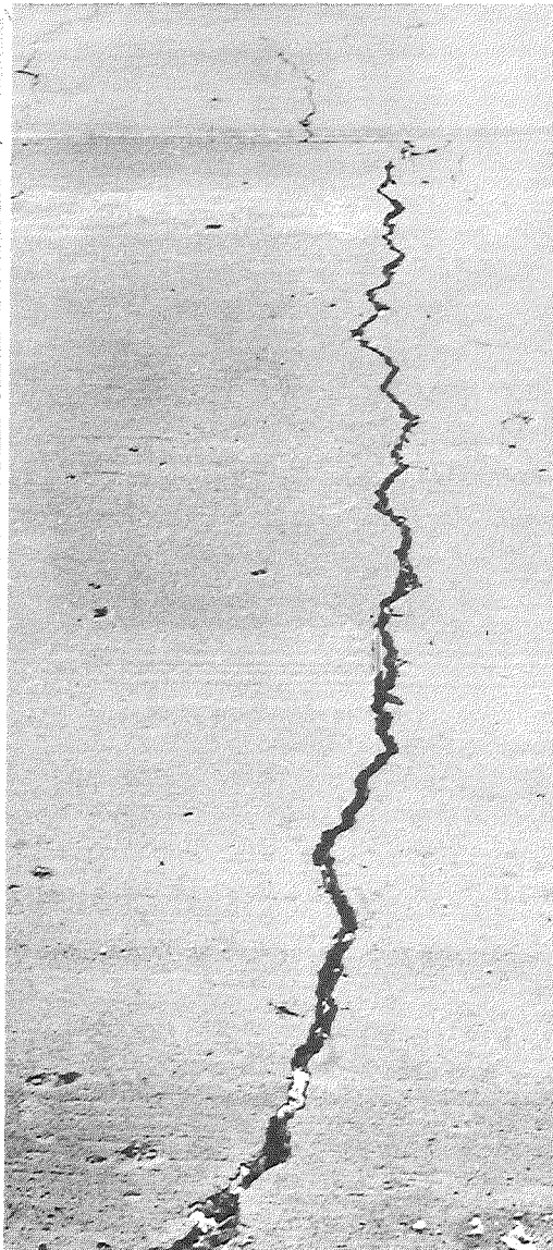
Sta 1045+75, westbound roadway (photo: January 1962)
