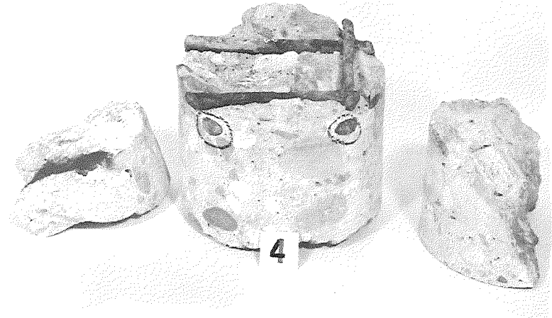
D. Core through traffic lane failure crack, indicating a Type 1 failure.
