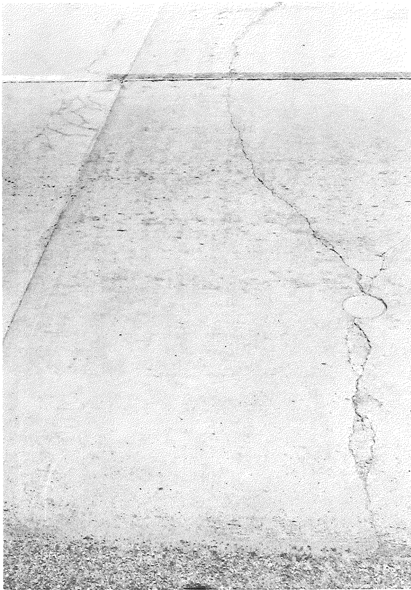
Sta 1044+66, eastbound roadway (photo: April 1960)
