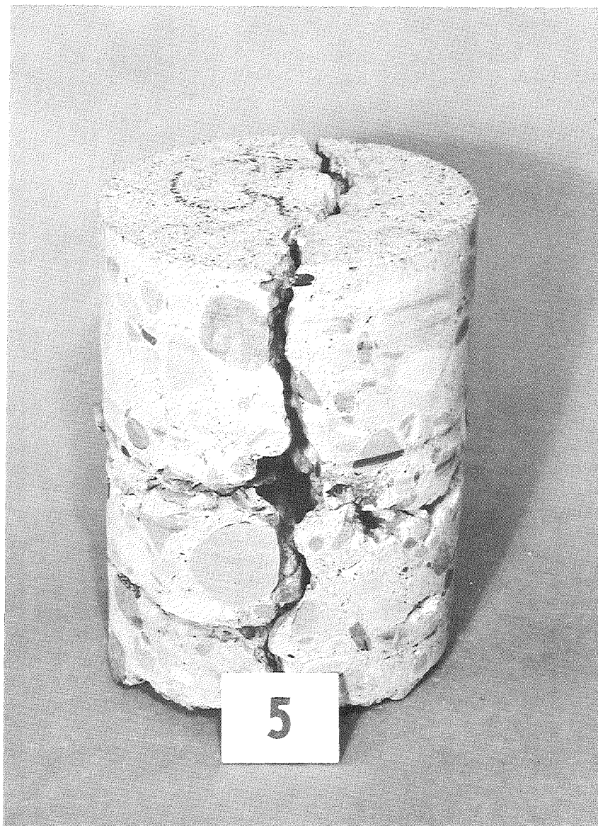
A. Core at failure crack, indicating a Type 2 failure.
